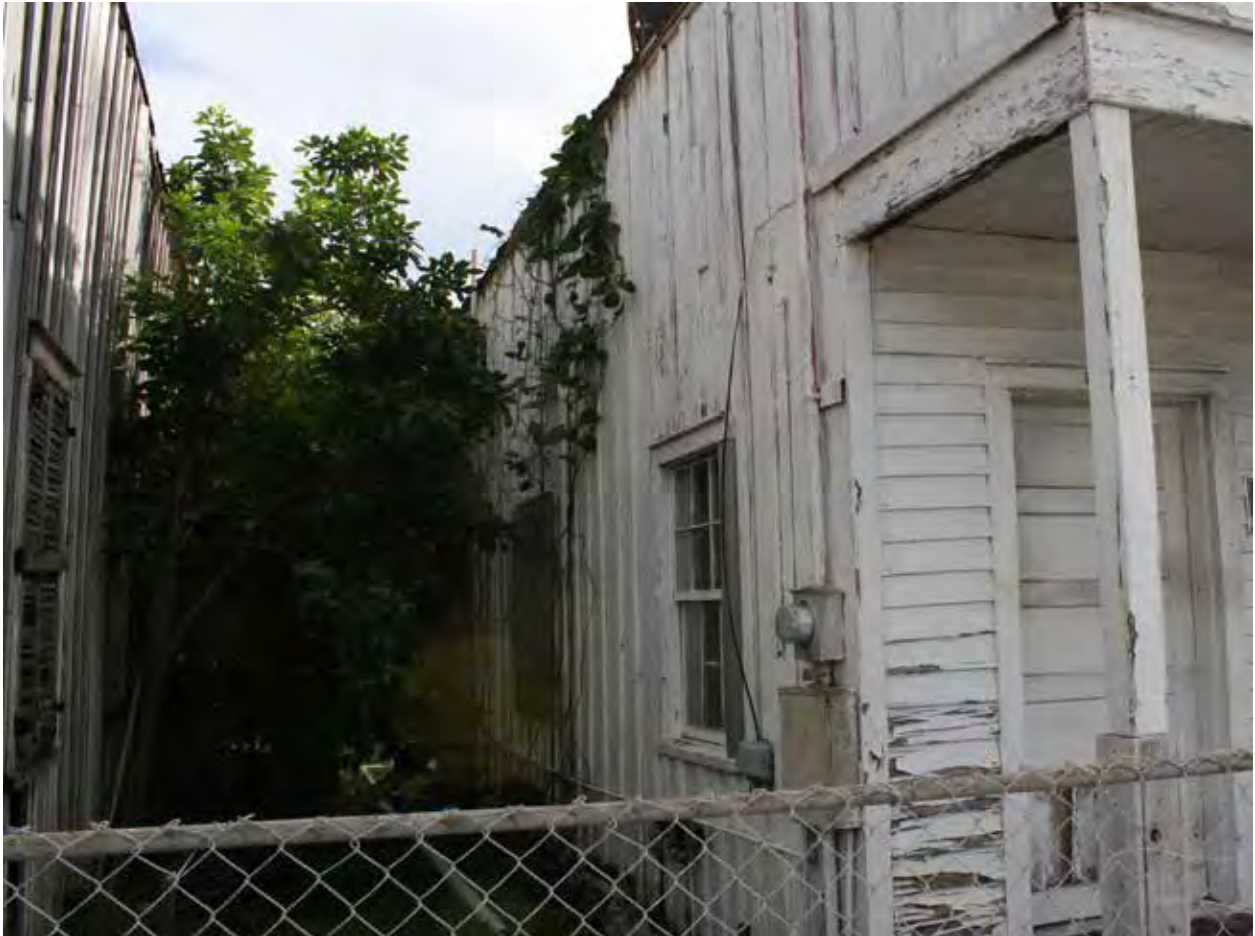
Side and Rear Façades
