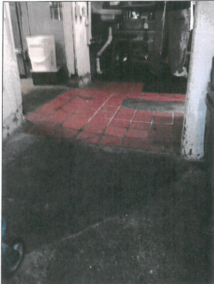
6.2 Picture 5 Typical Flooring Situation
