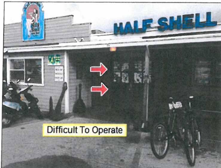
2.1 Picture 1 Front Door
