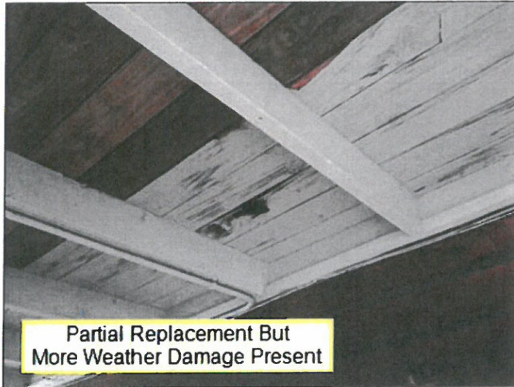
2.3 Picture 3 Front Porch Ceiling
