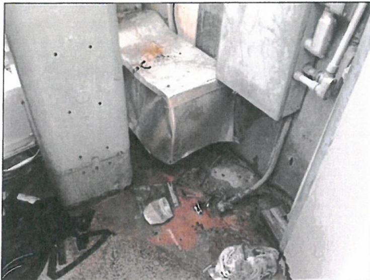
8.0 Picture 1 Service Entrance
