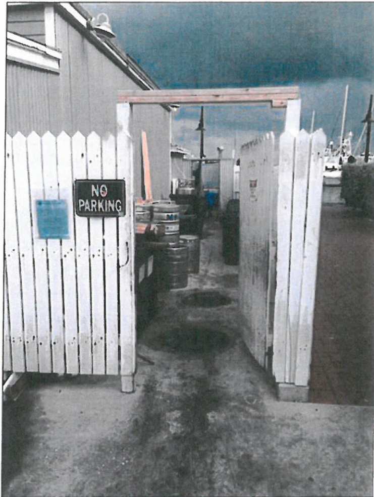
2.3 Picture 1 NE Side Of Building
