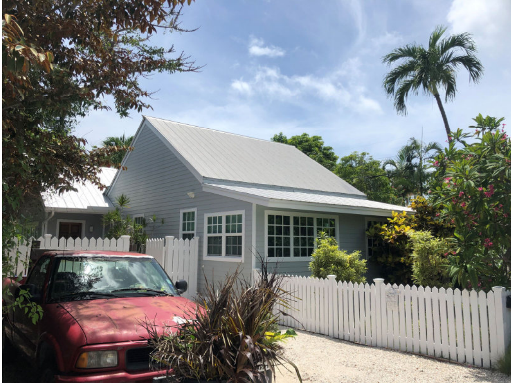
1310 Royal Street – Adjacent Property to North
