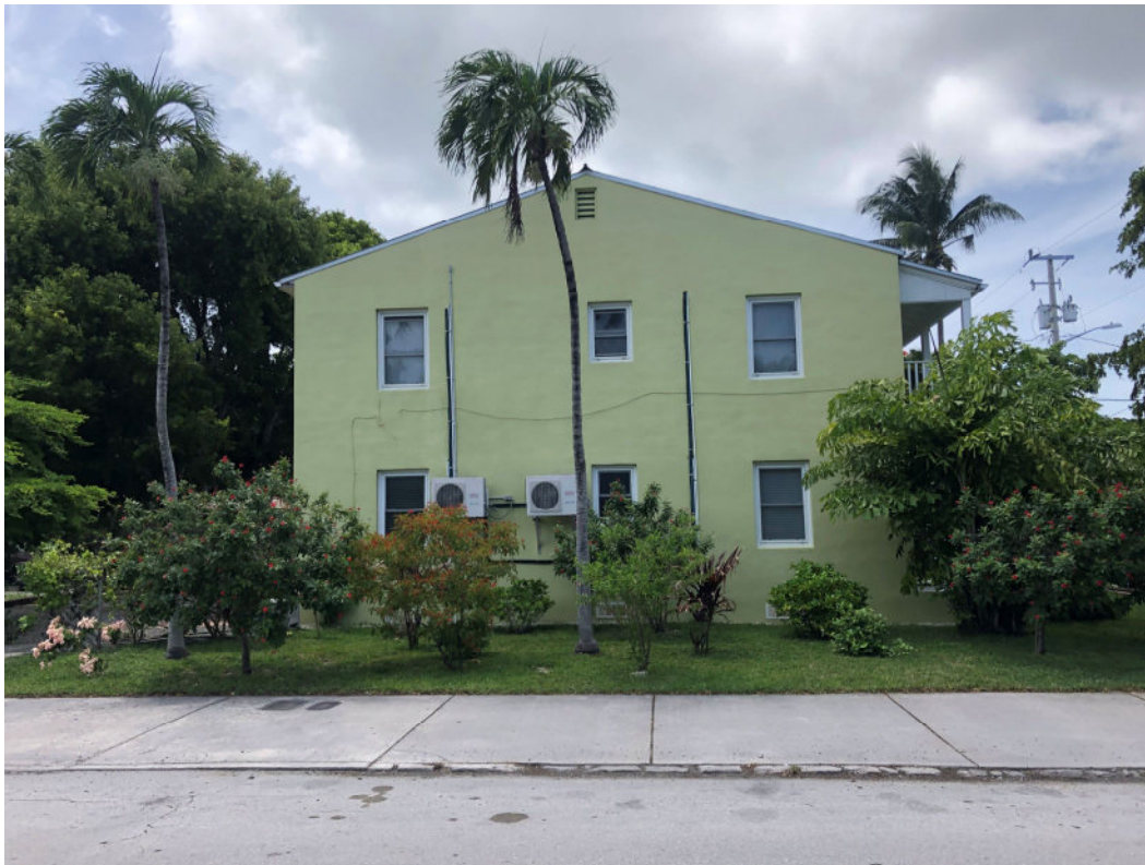
1320 Royal Street – View from South Street
