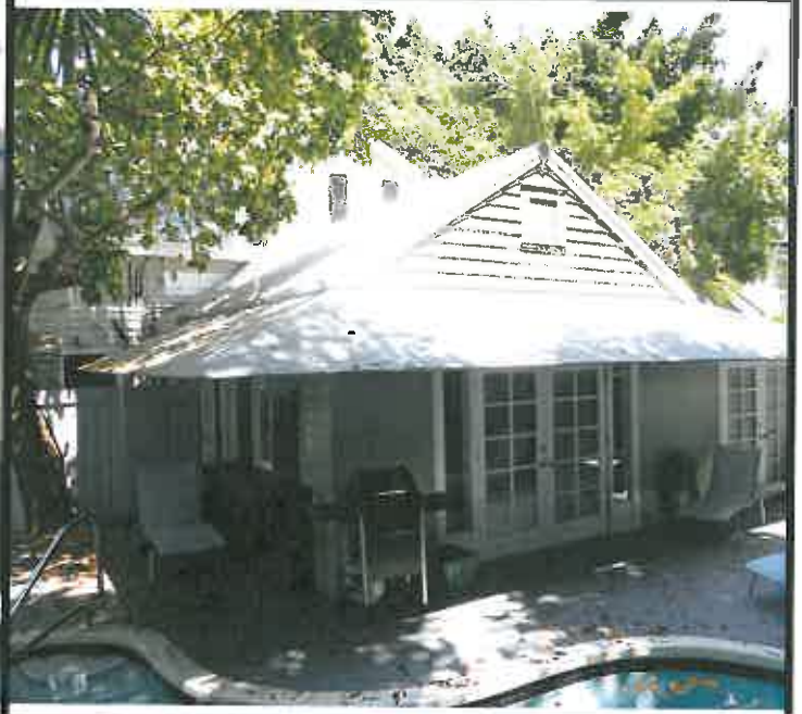
Exterior rear elevation looking at outdoor deck
