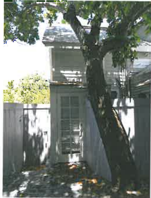
Existing bath and storage entrance.
