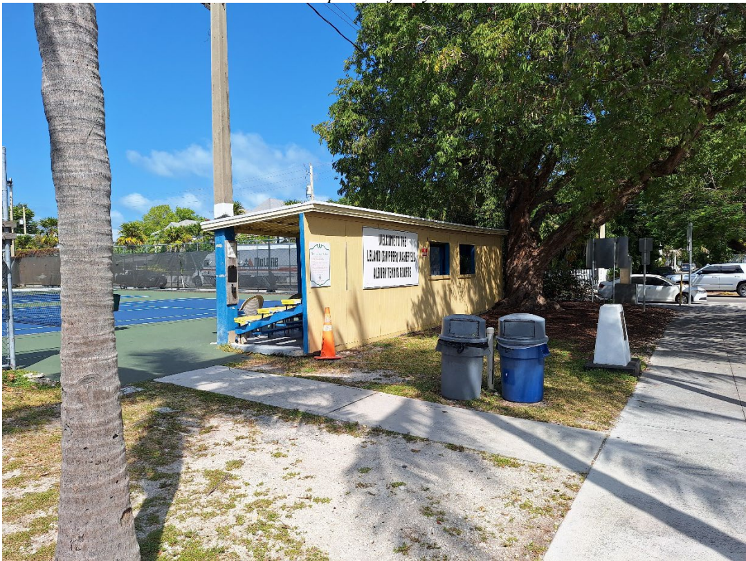
Current photo of property under review. (existing shade structure)
