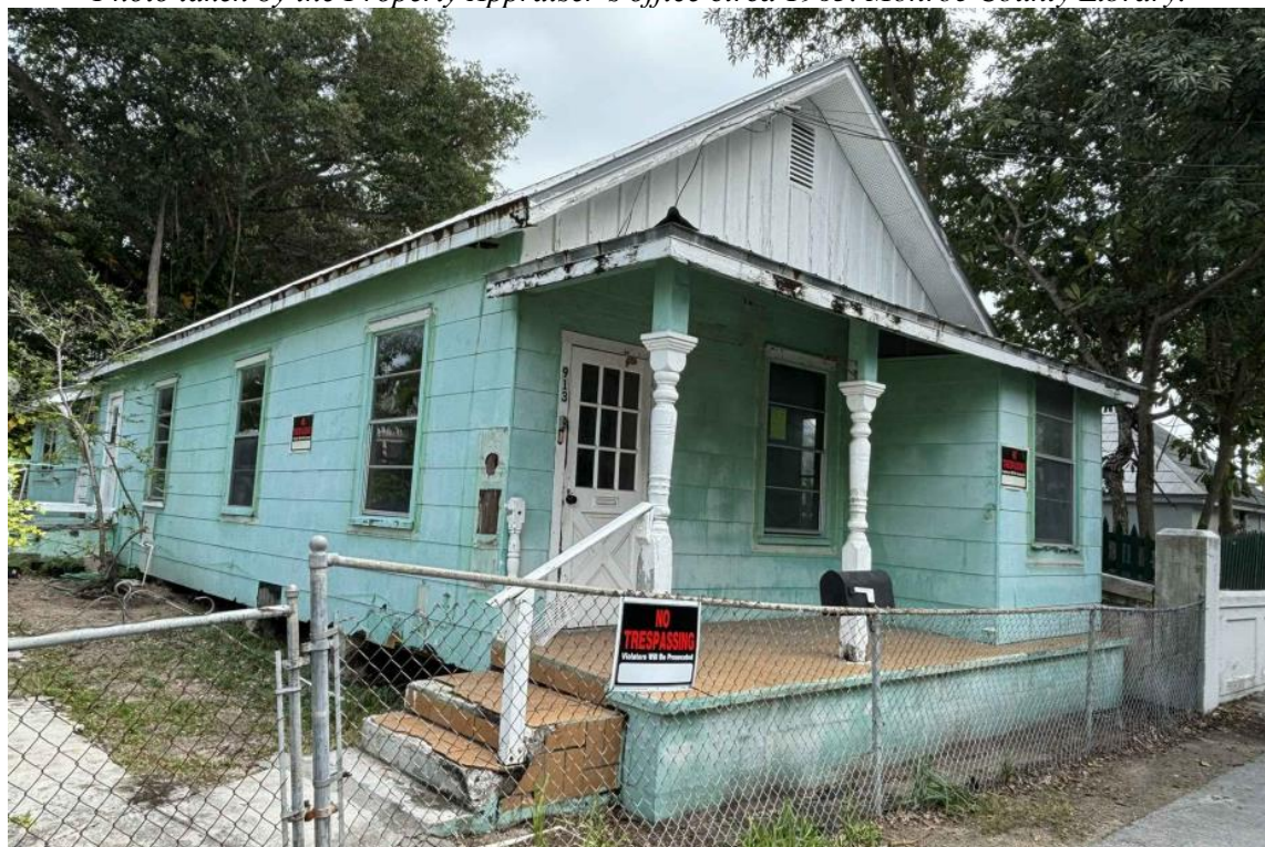
Current photo of house under review.
