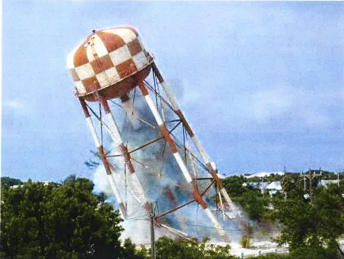
Water Tank Demolition, NAS Key West
