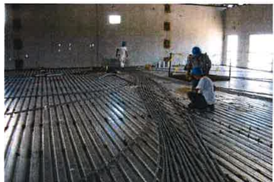
Slab Rough-In, Marathon High School
