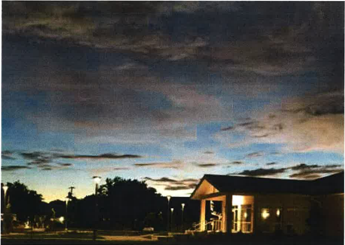
Marathon City Hall - New 15,000 SF Municipal Building, Marathon, FL
