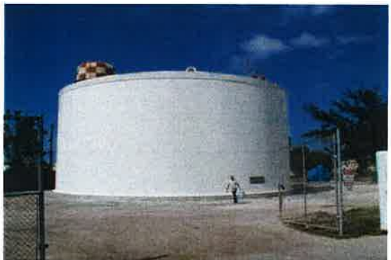
700,000 Gallon Concrete Water Tank
