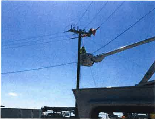
Installing Guy Wire NAS KW
