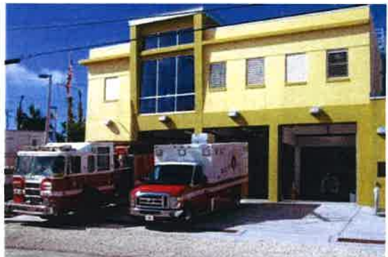
Conch Key Fire Station, Conch Key, FL
