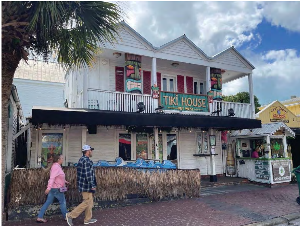
Current conditions at front elevation.
