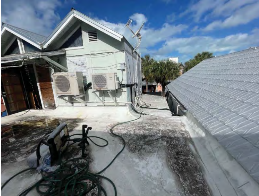
Current conditions at roof deck
