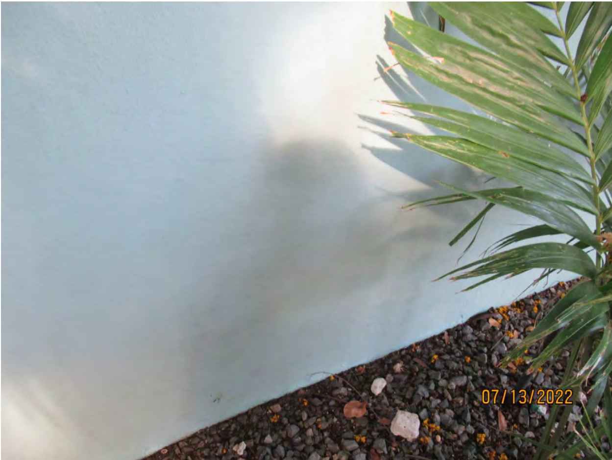
Photo of structure wall near tree.
