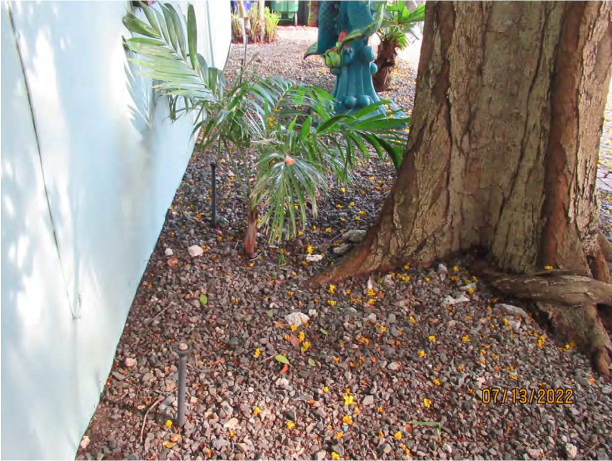
Photo of base of tree showing distance from tree to foundation, view 1.
