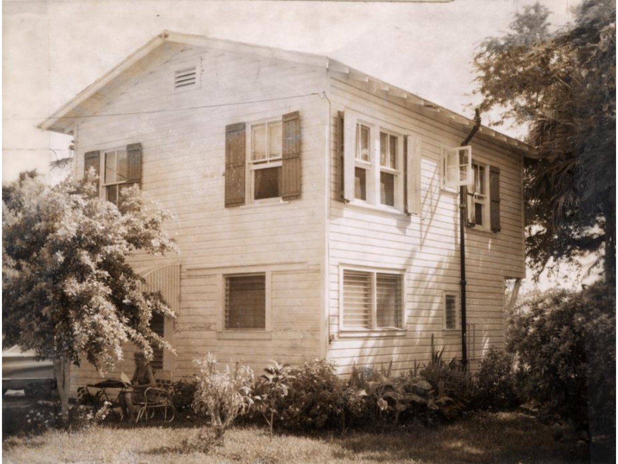
1965 photo showing the structure at 1319 Elizabeth Street.
