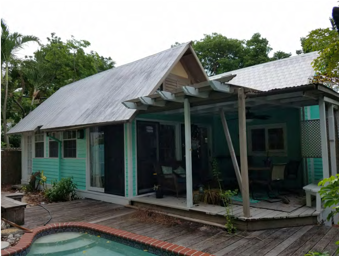
Side (west) façade. Note: this addition was constructed after 1968. Replace all doors and windows with painted wood units. New bifold doors. Repair existing porch roof. New wood decking.
