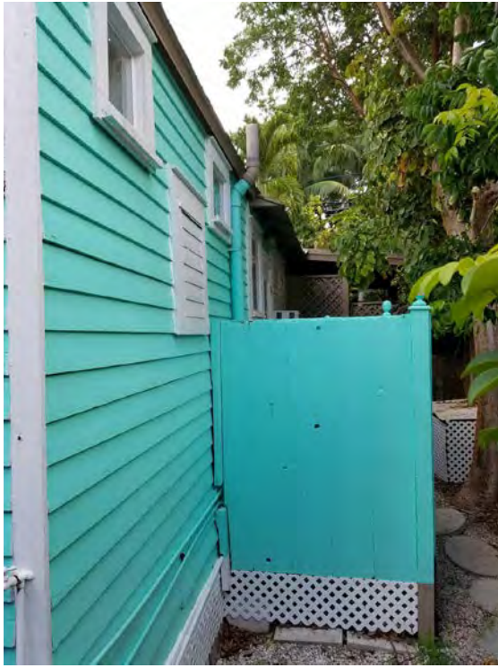
Side (east ) façade.
