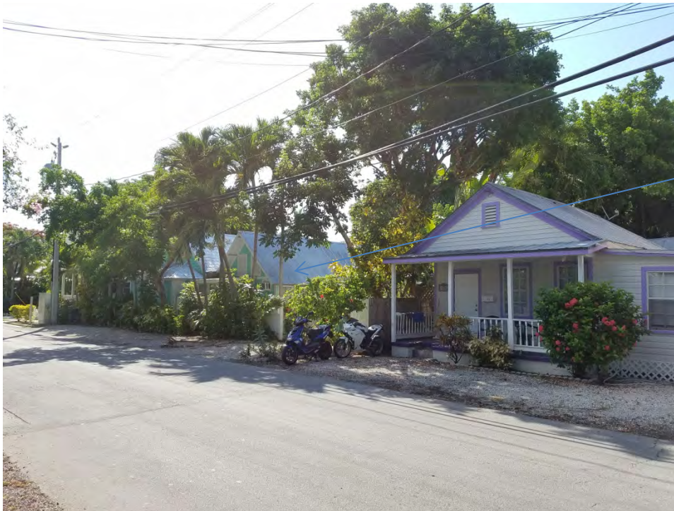
Street view from west side.
