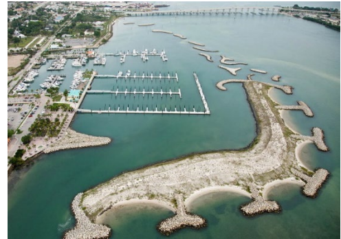
Fort Pierce Storm Protection Island, Tetra Tech
