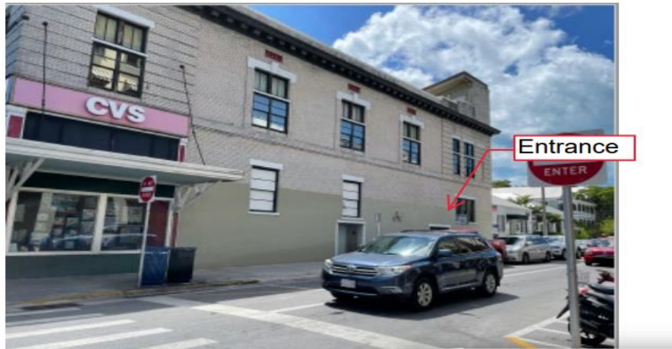
Street View of Receiver Site
