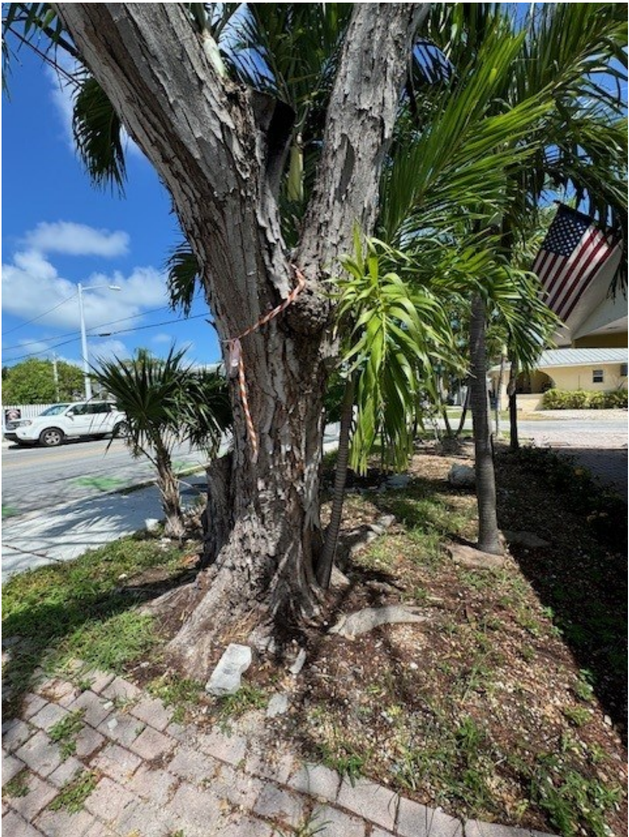
The trunk and limbs of this tree have been destroyed by flat-headed borer and subterranean termites.
