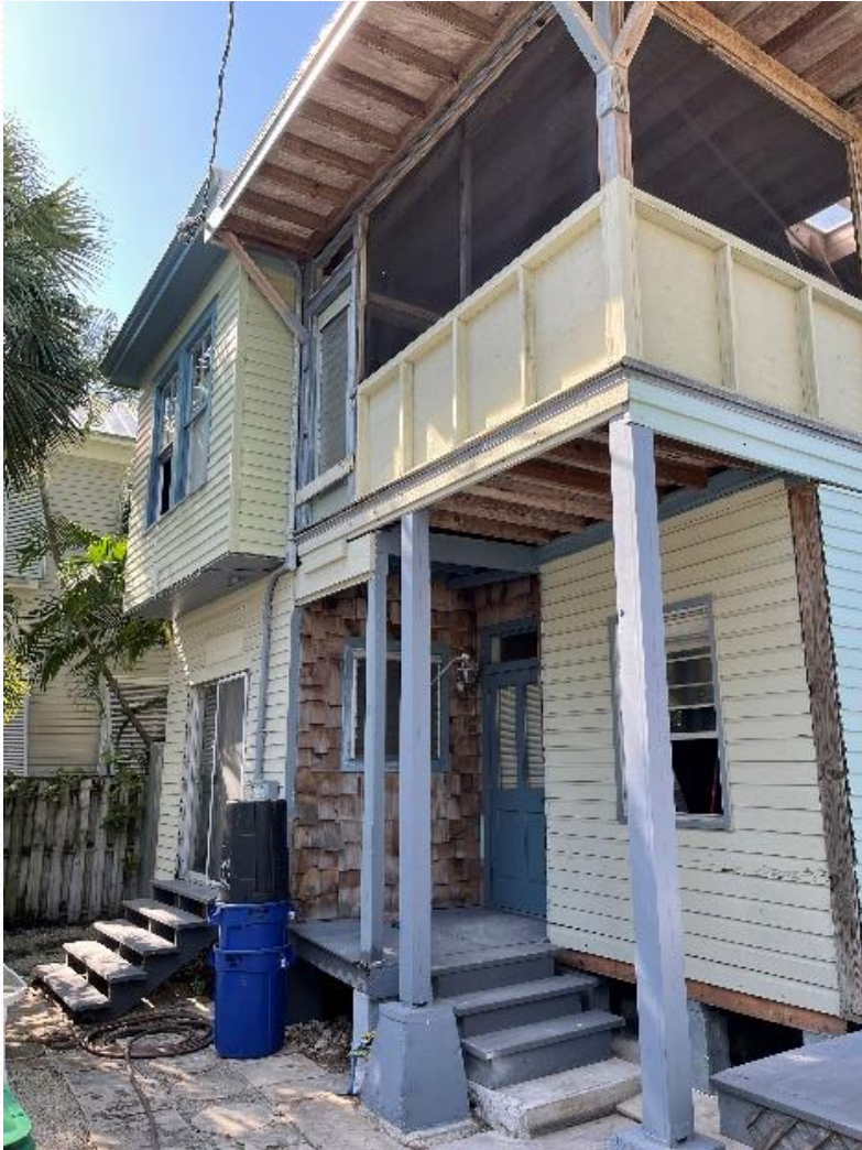
Prior to Lift
