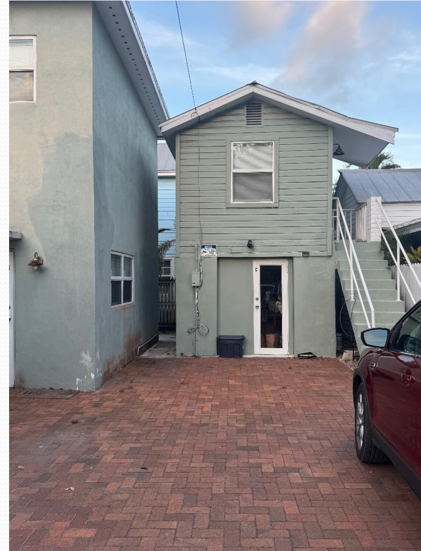
Off of Whitehead Street- extended roof overhang
