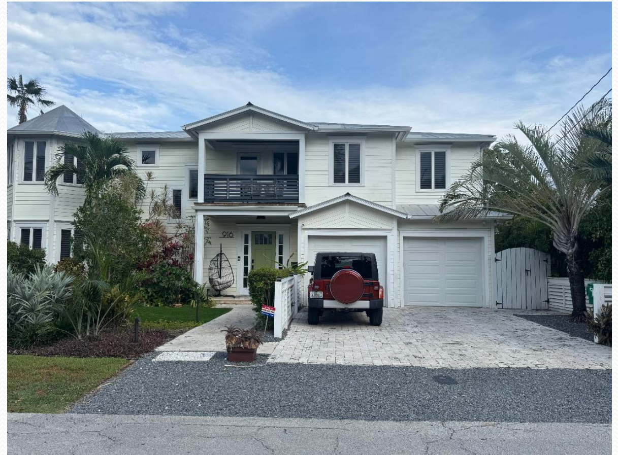
916 Washington Street, Attached to house
