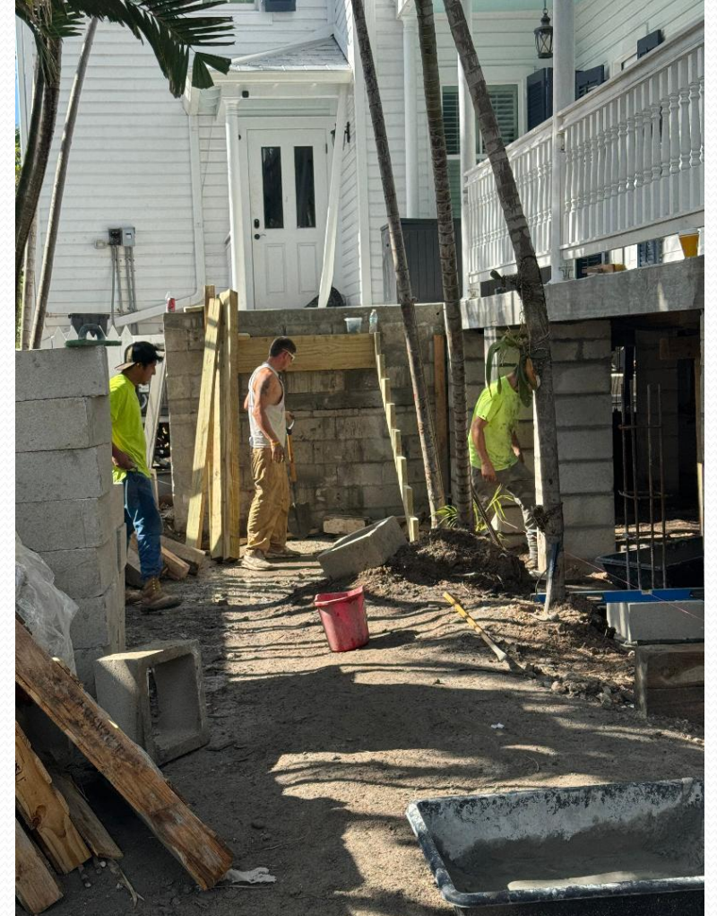
408 United...Done 2000, attached garage to house!
