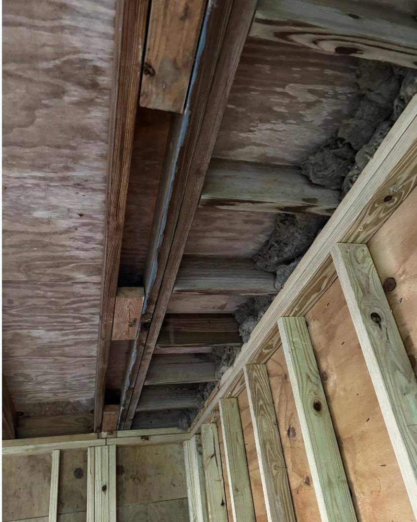
East Joist addition 1975+ Inside
