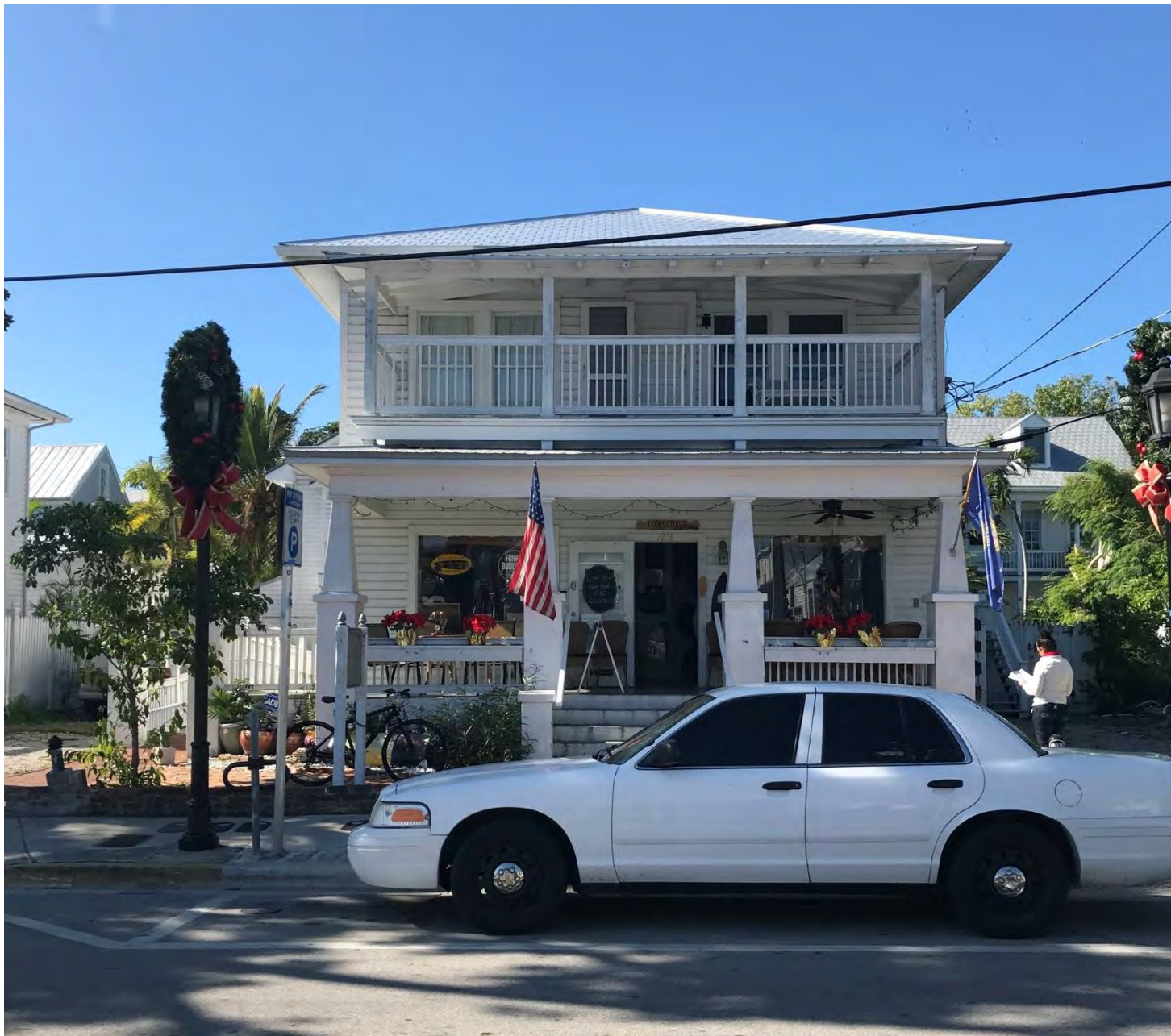
1218 Duval Street FRONT VIEW
