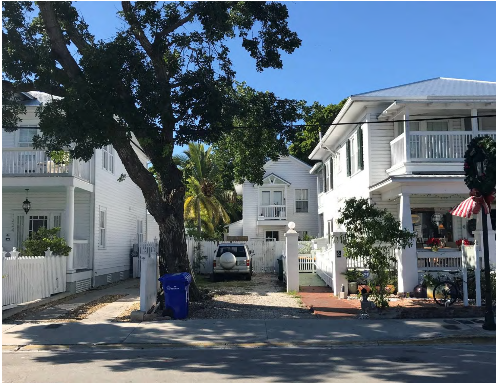
1218 Duval Street FRONT VIEW
