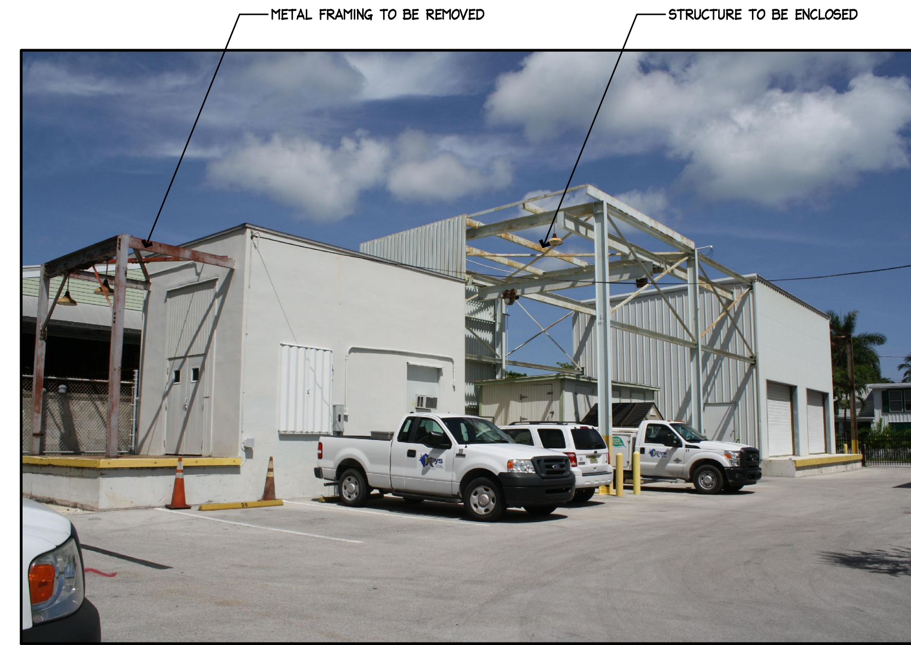
6 PHOTO OF EXISTING STRUCTURE A6.3 N.T.S.
