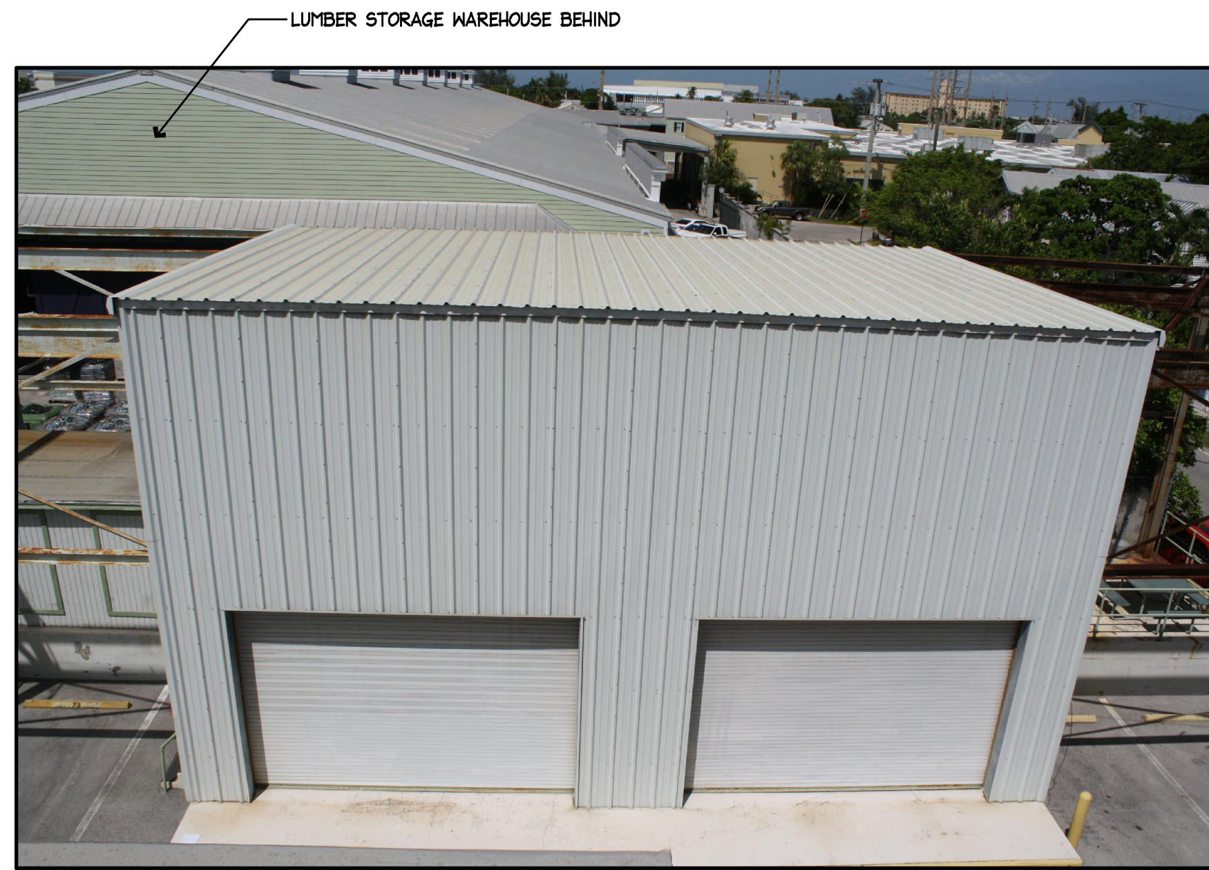
8 PHOTO OF EXISTING STRUCTURE A6.3 N.T.S.
