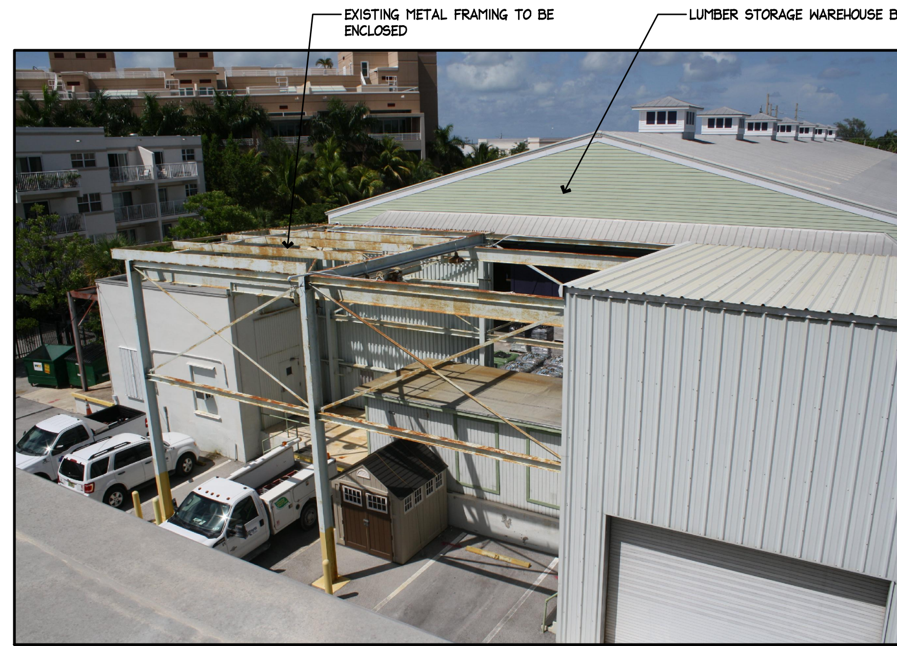
7 PHOTO OF EXISTING STRUCTURE A6.3 N.T.S.
