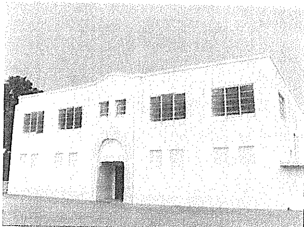
Exterior view of Gymnasium (Building D)
