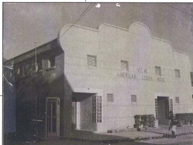
HISTORIC PHOTO OF FRONT OF BUILDING. NOTE GLASS BLOCK AROUND DOOR OPENINGS. CONTRACTOR SHALL CAREFULLY REMOVE EXISTING STUCCO, AS GLASS BLOCK MAY STILL EXIST THERE. ARCHITECT TO INSPECT AREA DURING AND AFTER DEMOLITION. IF GLASS BLOCK IS FOUND, IT SHALL BE RESTORED. IF NO GLASS BLOCK IS FOUND, CONTRACTOR SHALL REPLACE GLASS BLOCK PER PHOTO. FOR BIDDING PURPOSES, CONTRACTOR SHALL ASSUME THAT GLASS BLOCK SHALL BE REPLACED.
