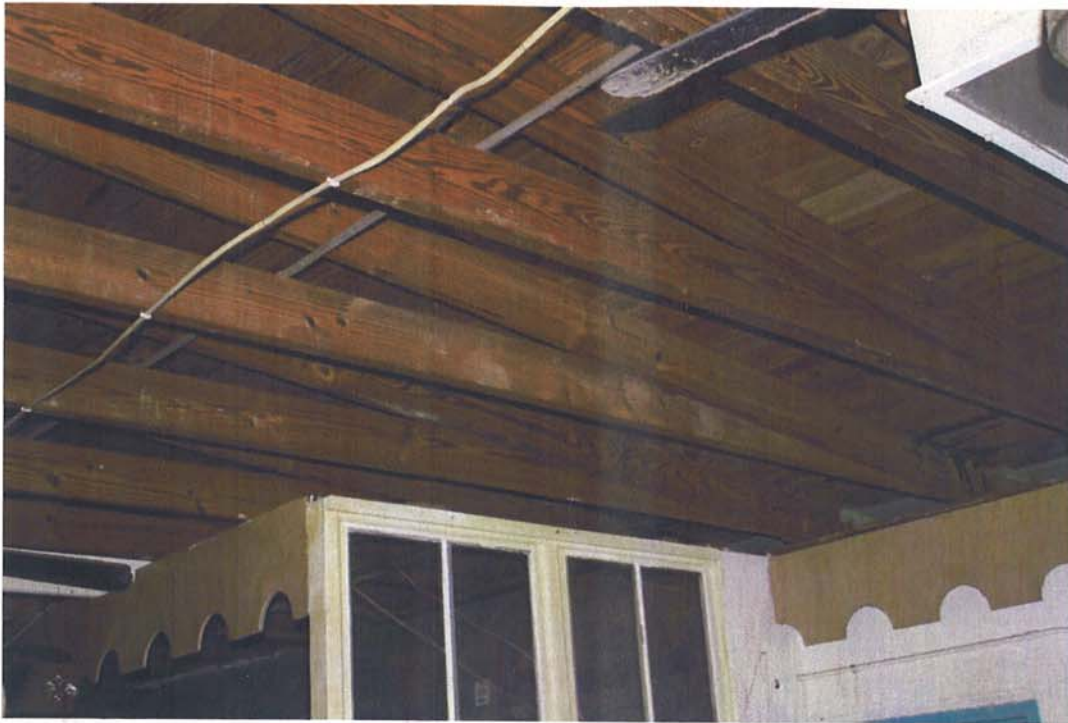
Photo of ceiling at kitchen. Sister roof rafters per Structural drawings.
