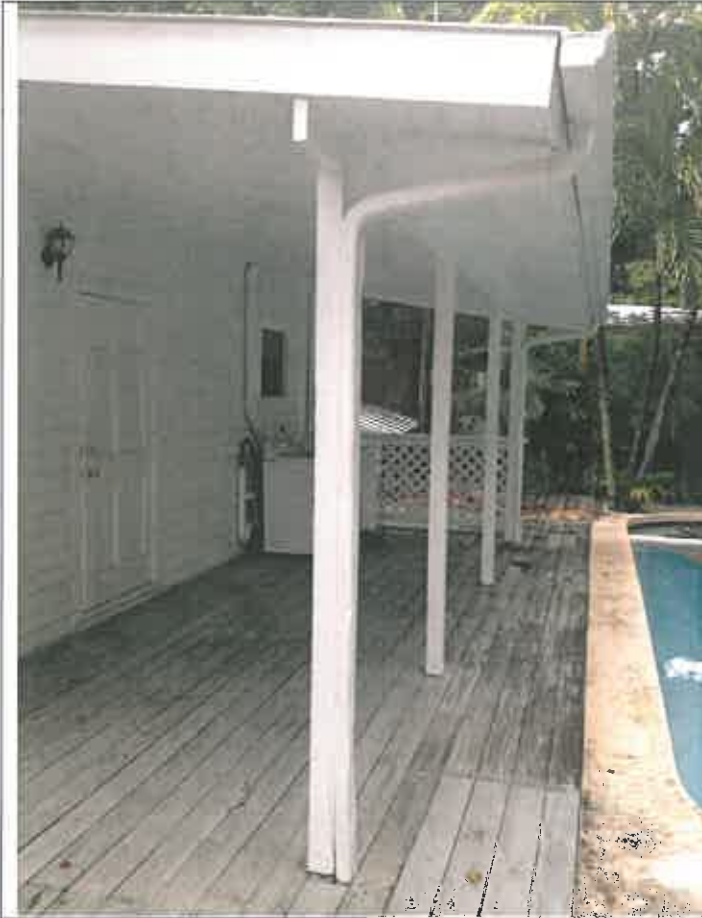
1008 Watson – Covered Rear Deck
