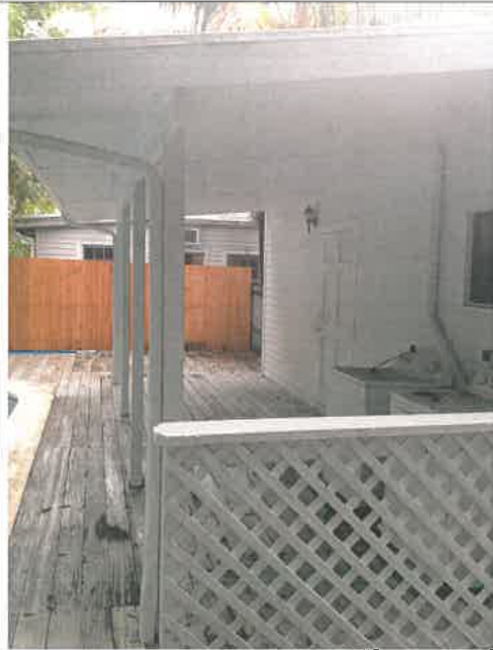
1008 Watson – Covered Rear Deck
