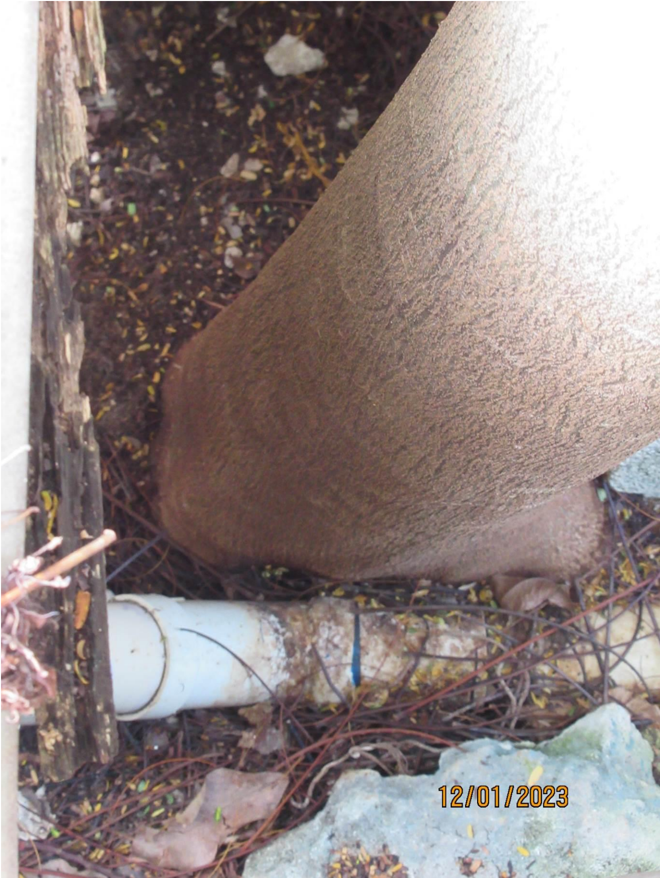
Close up photo of base of tree.
