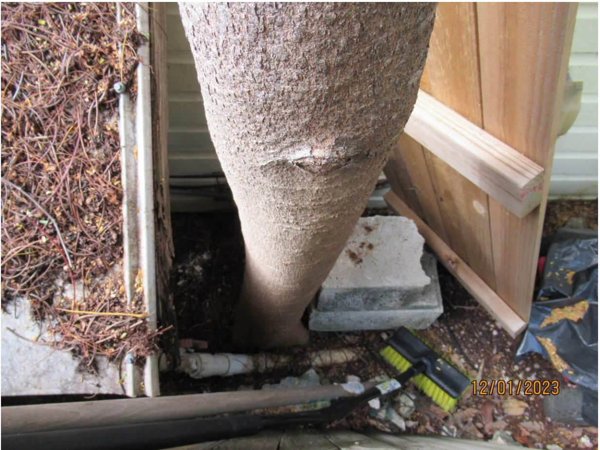
Photo showing location of base of tree, view 1.
