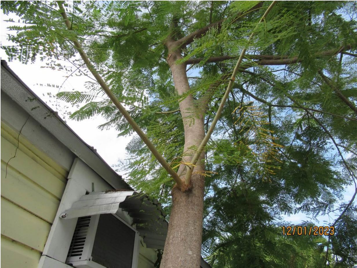
Photo of tree trunk and canopy in relation to structure, view 1.
