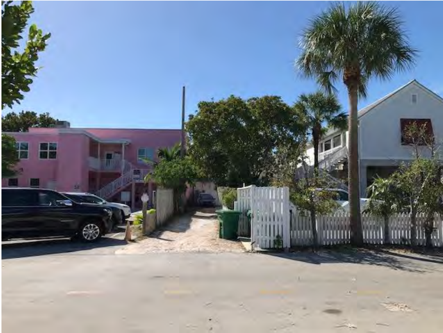
619 Duval Street REAR VIEW
