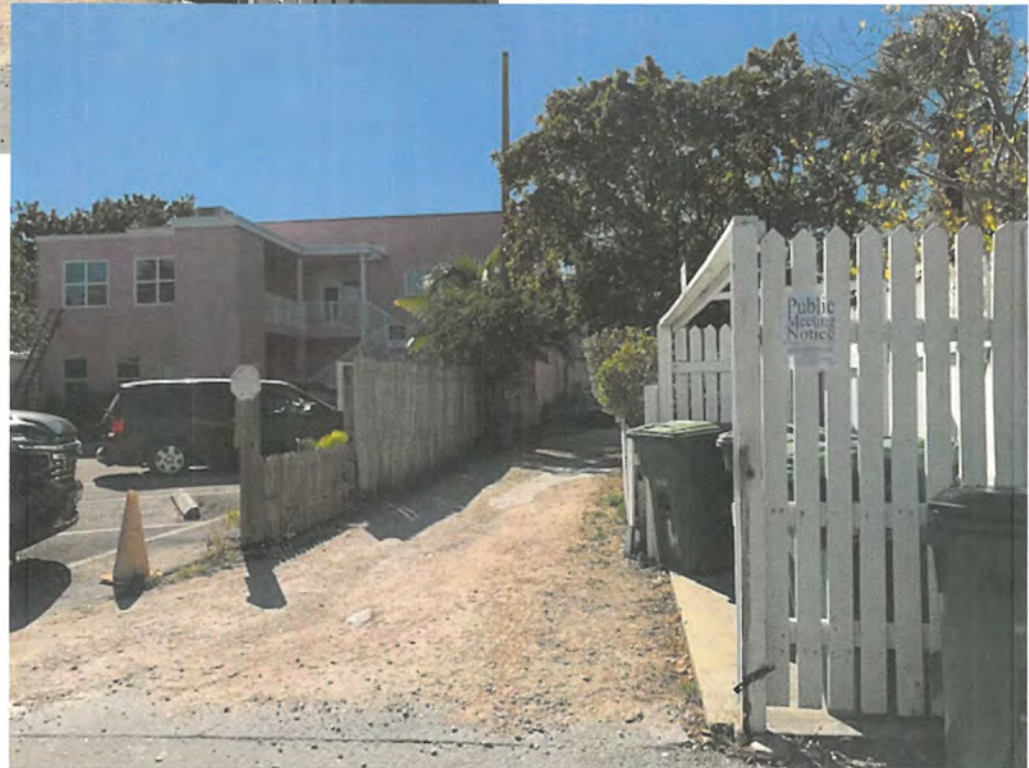
619 DUVAL STREET REAR VIEW
