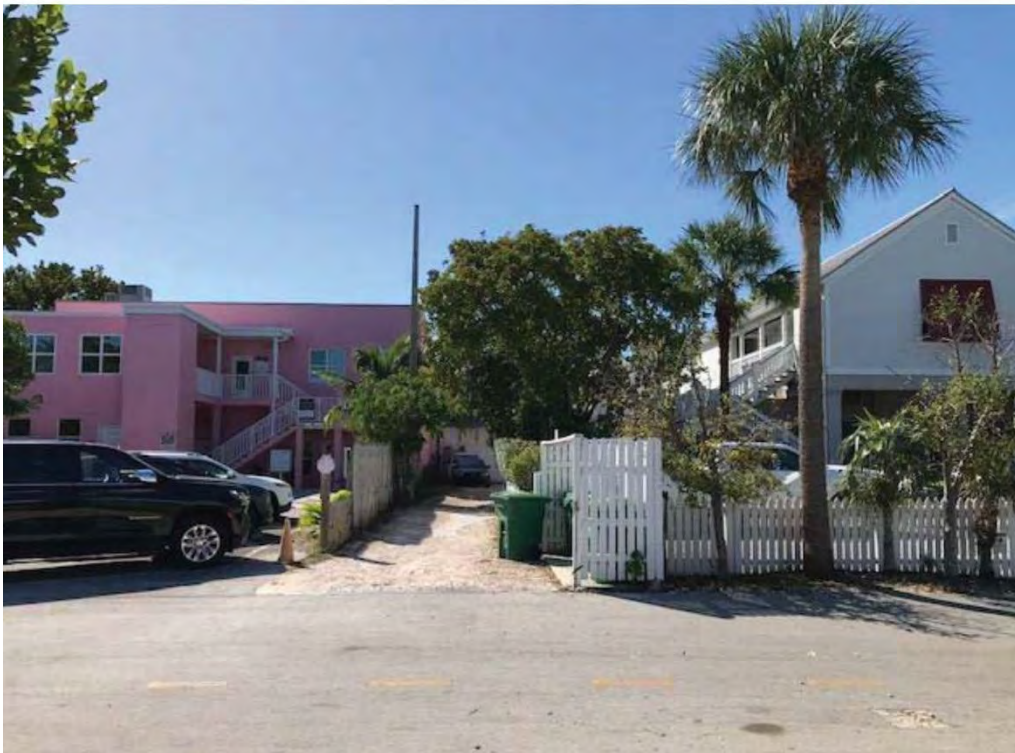
619-621 Duval Street rear elevation.
