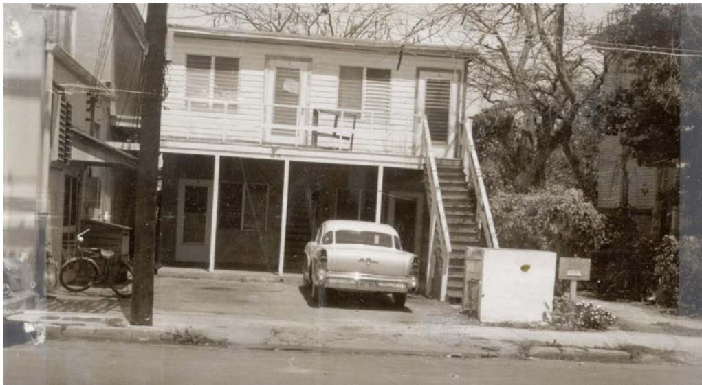
Photo of 1205 Virginia Street circa 1965, in front of building under review before gabled roof with dormer was added.
