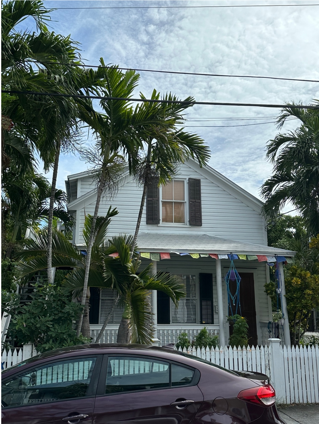
1210 Virginia Front View from Virginia St. showing Shed Dormer
