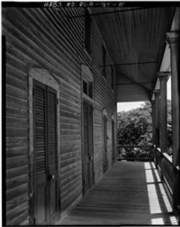
View of 2 nd floor porch, date unknown, but probably 1967. Note traces of paint.
