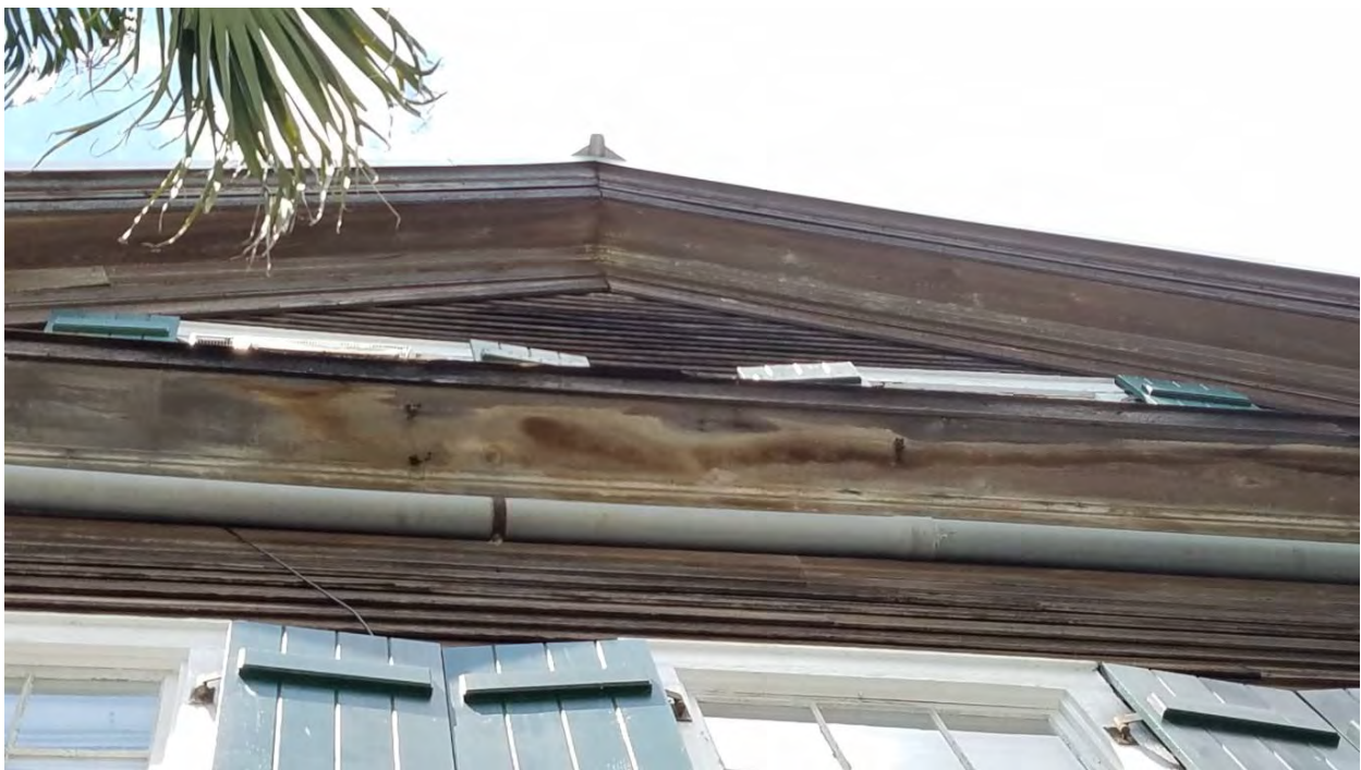
Detail view of east gable. Note traces of paint at fascia.
