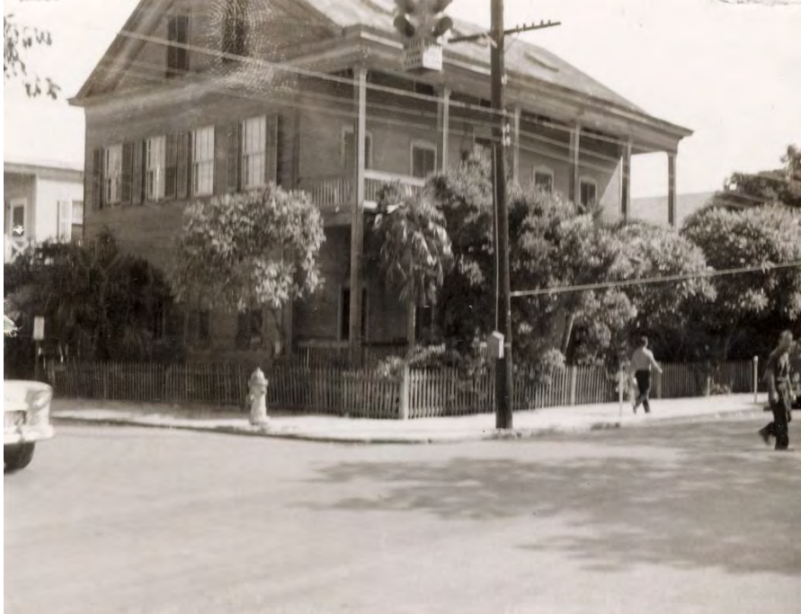
View of SW corner, 1965.
