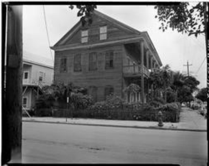
View of west façade, ca. 1933.
