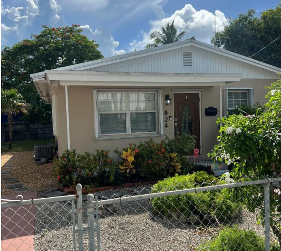
Current photo of house under review.
