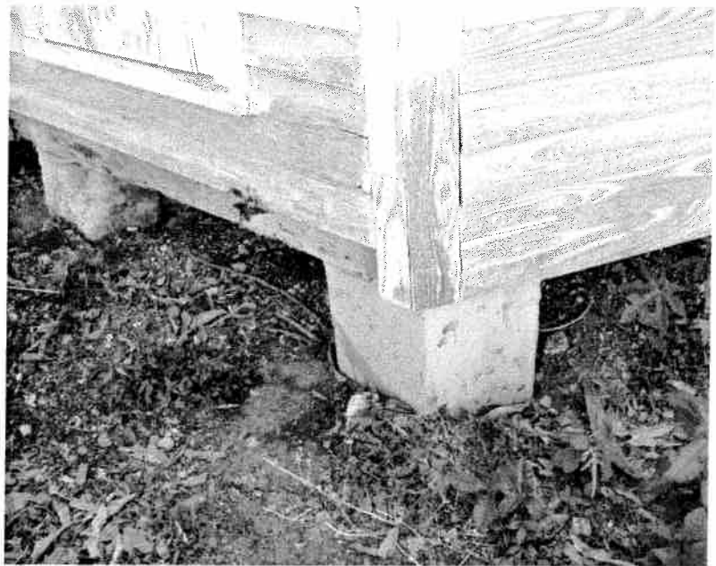
Figure 17 Foundation Piers
