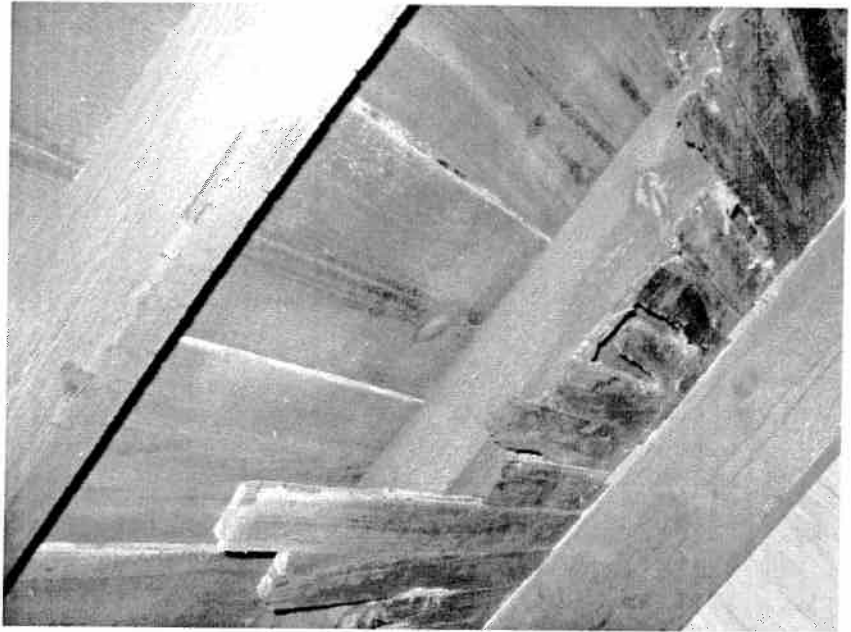
Figure 59 Evidence of 1964 Fire
