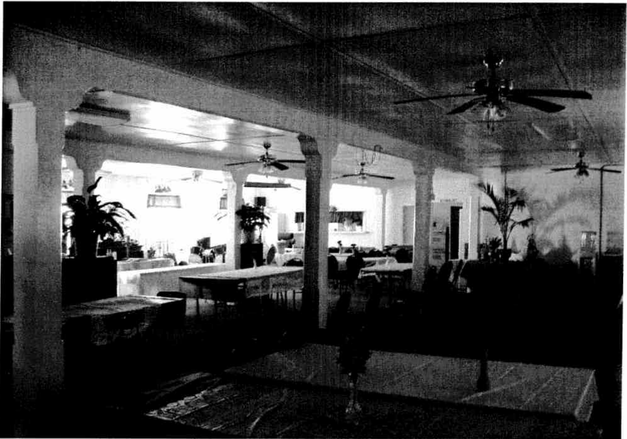
Figure 62 First Floor Interior Lights
