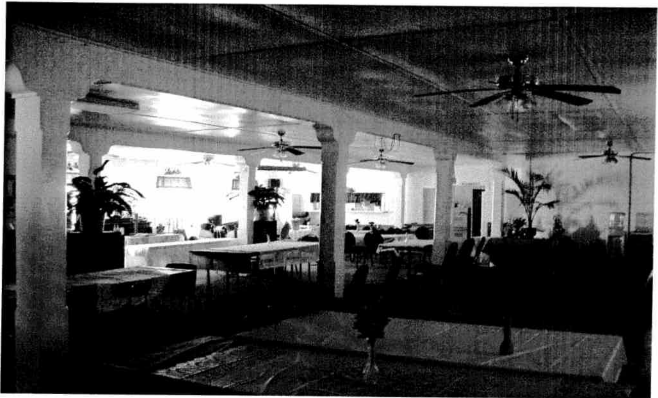
Figure 24 Second Floor Supporting Columns (View of Fellowship Hall)
