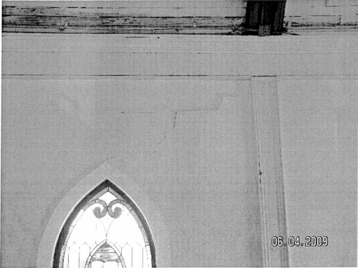
Nave wall, North
