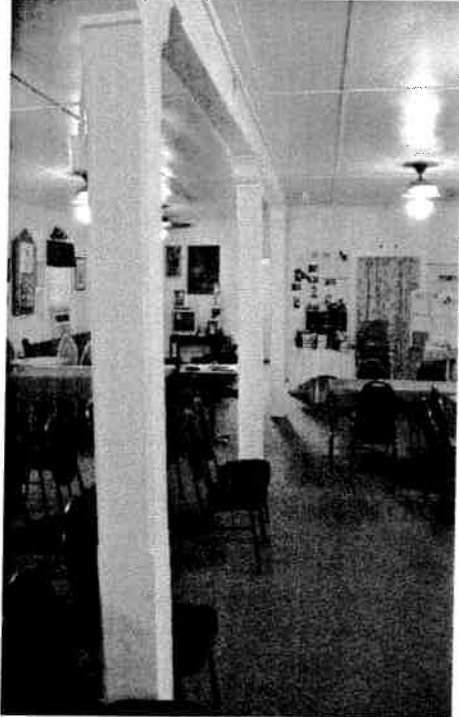
Figure 15 Racked Columns
