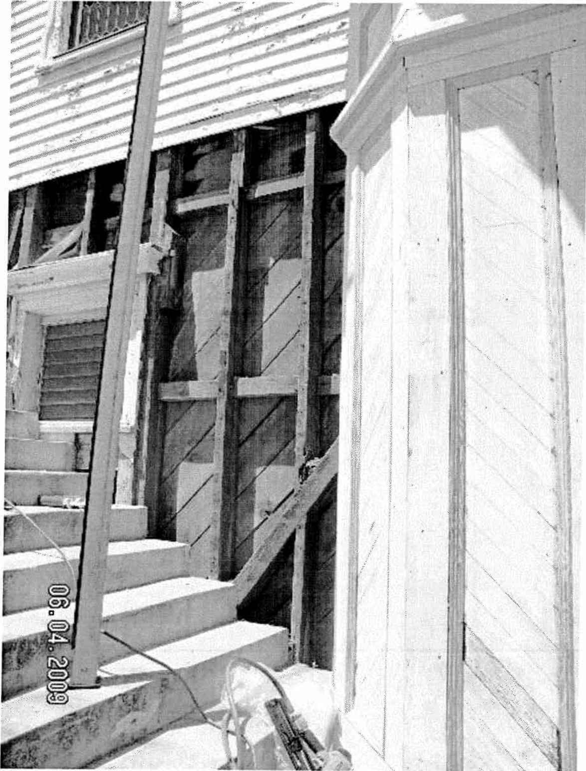
Front wall by entrance.
