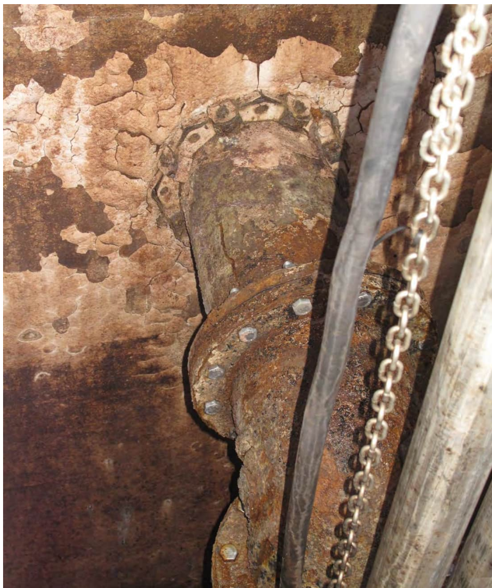
Wet well failed liner
