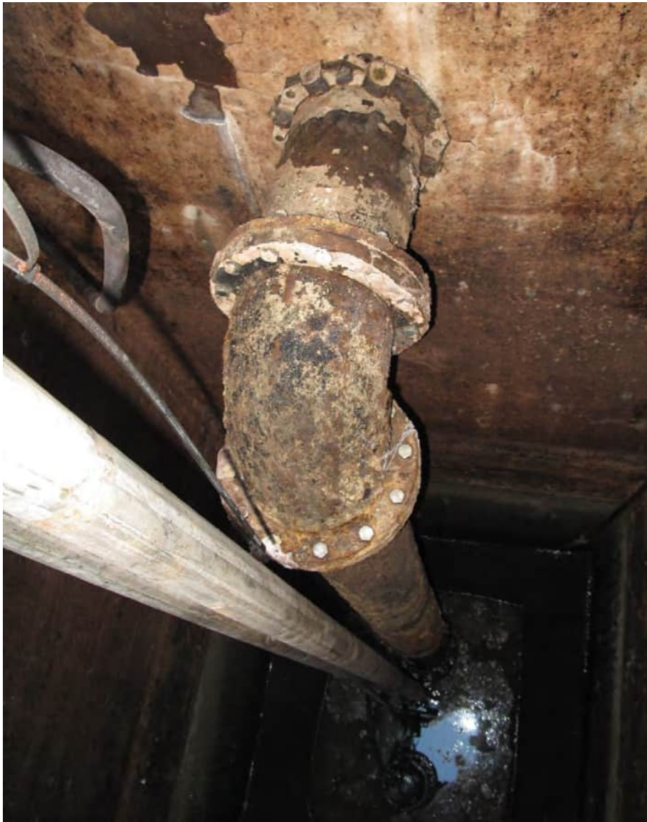
Wet well liner failing
