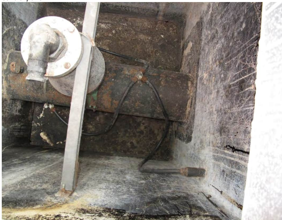
Flowmeter vault with air release valve
