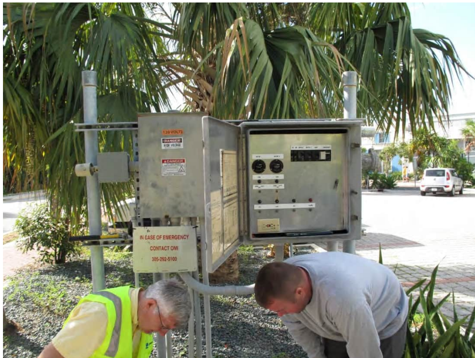
Pump control panel and main disconnect
