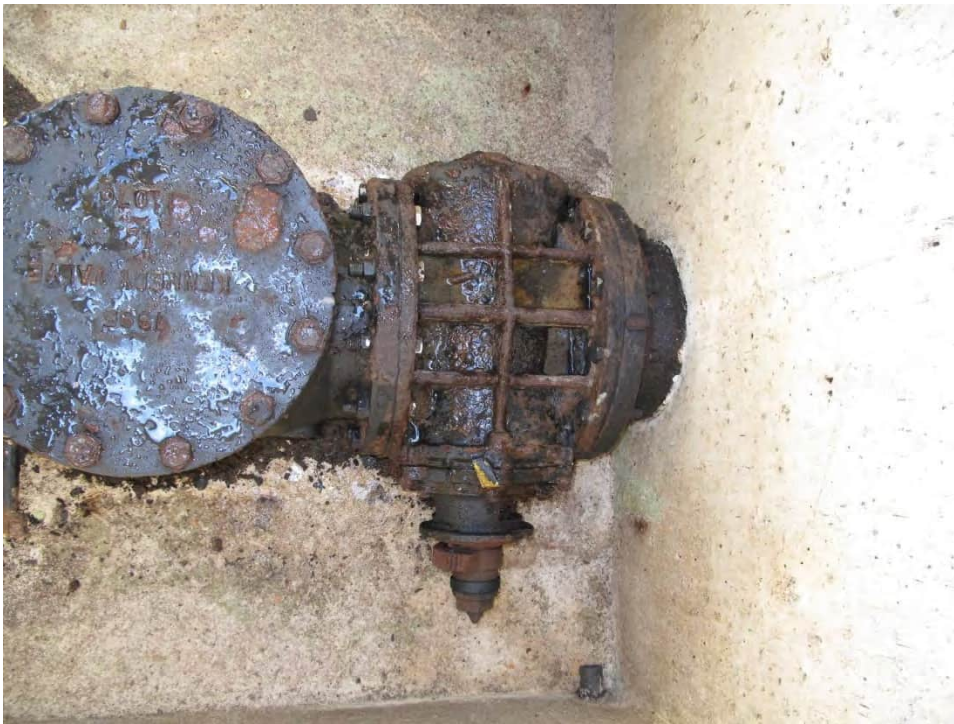
Corroded valve in valve vault
