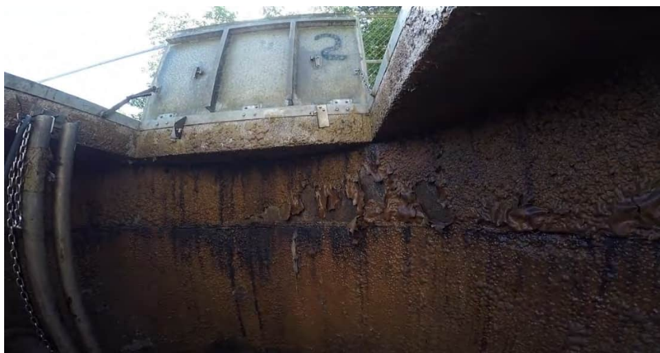
Failed liner in wet well
