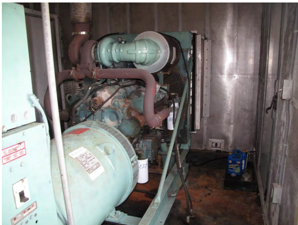
Emergency generator inside enclosure
