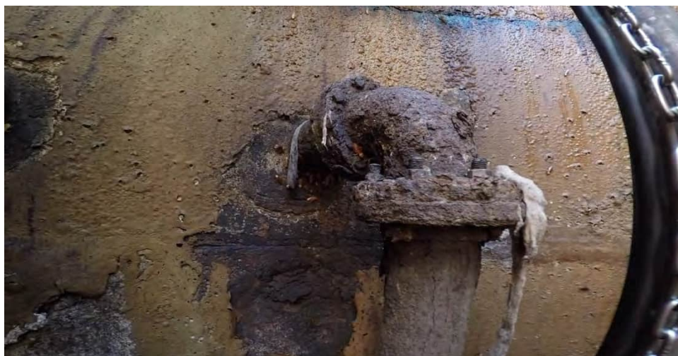
Corroded pipe in wet well
