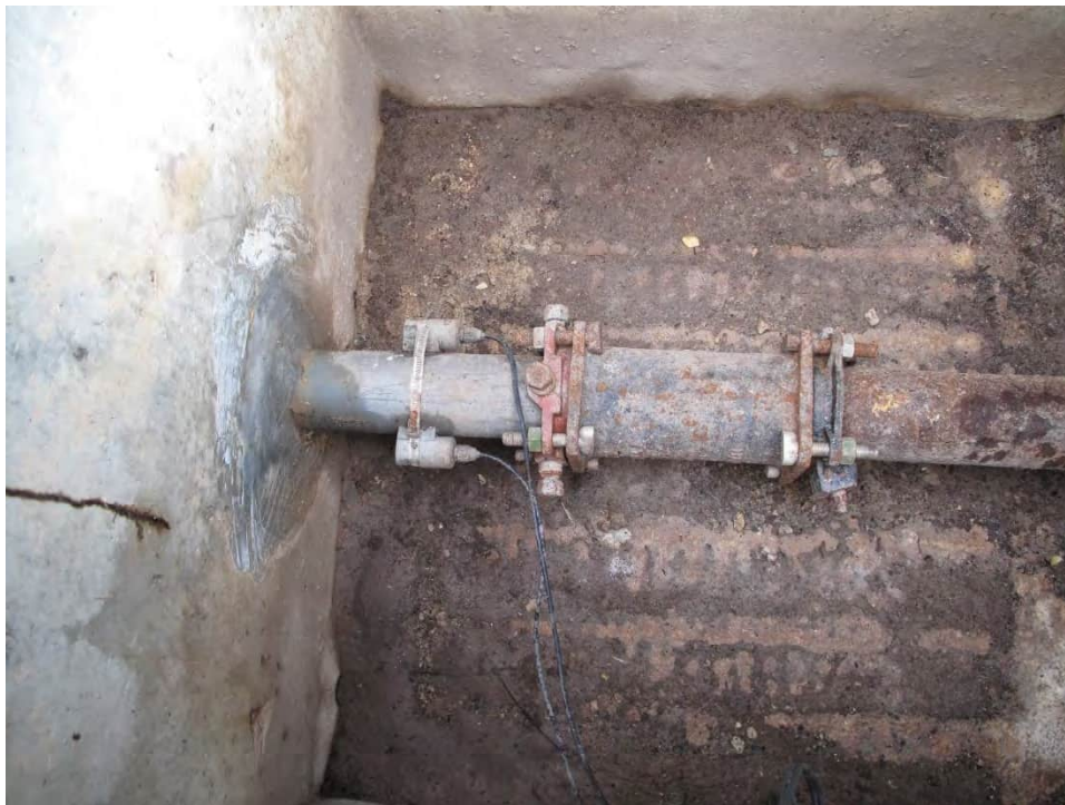
Flowmeter vault with failing pipe
