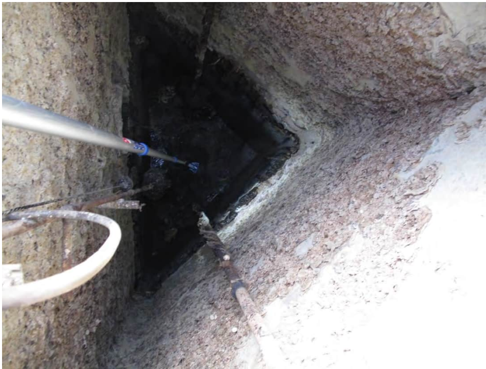
Failing concrete in splitter structure
