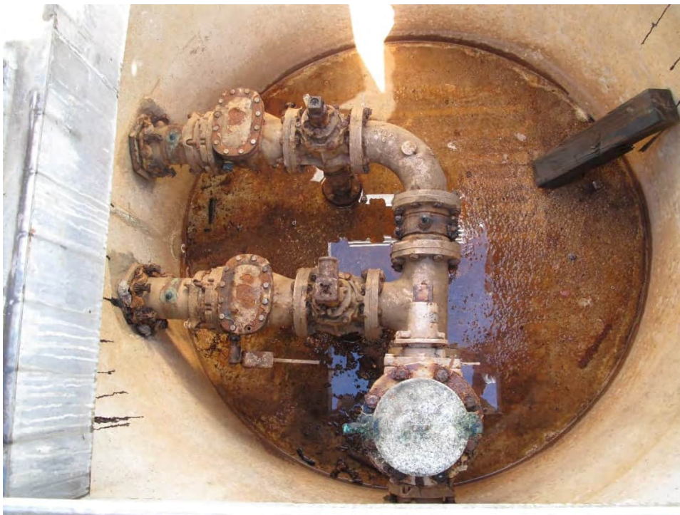
Valve vault with bypass pumping connection
