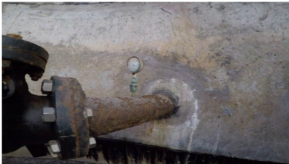
Corroded pipe in valve vault
