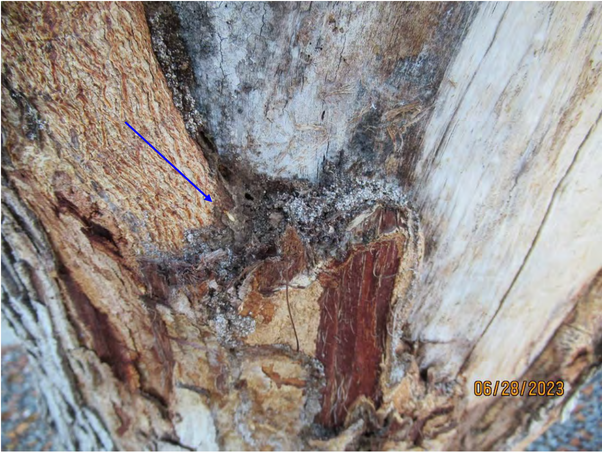
Close up photo of trunk damaged area showing dead wood and subterranean termite and trail, view 3.
