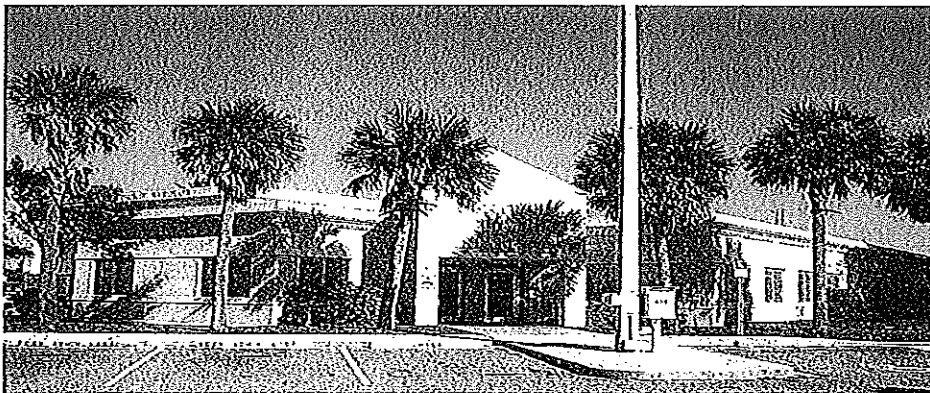
Key West Central Fire Station
