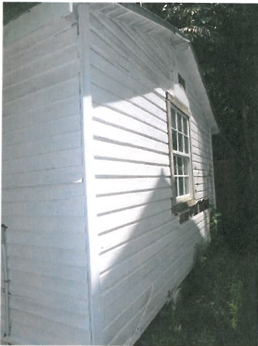
View of the rear of the secondary structure
