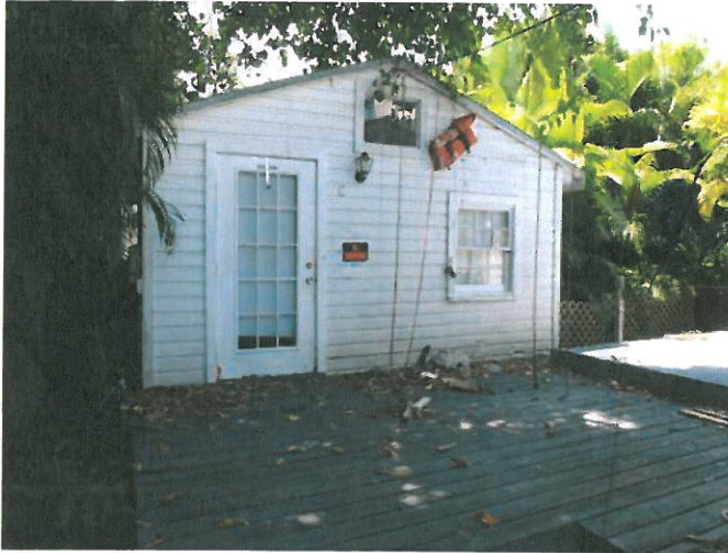
View of the front of the secondary structure behind the main structure
