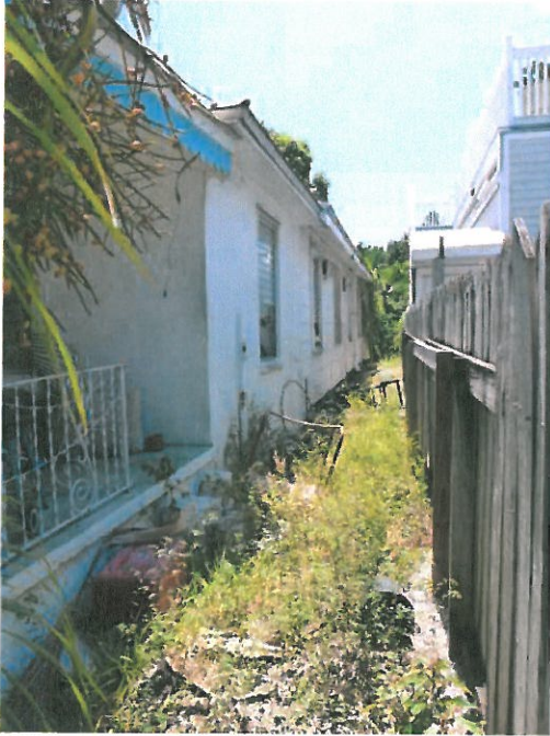
View of west side of main structure
