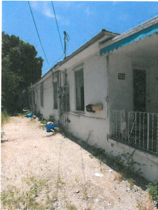
View of east side of main structure
