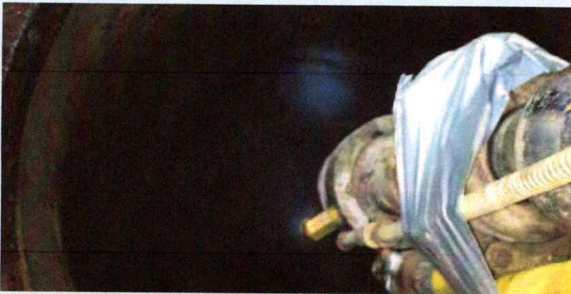
Spin head applying GeoSpray manhole lining.
