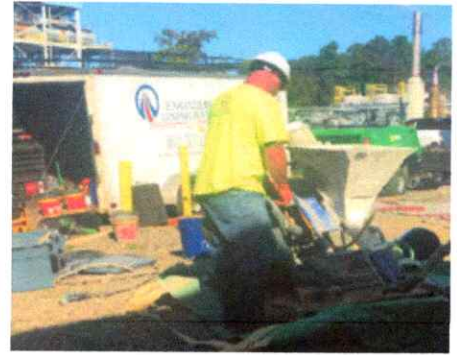
Equipment set up for manhole repair.
