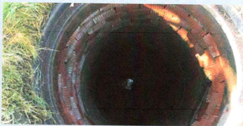
Brick manhole prior to rehabilitation.
