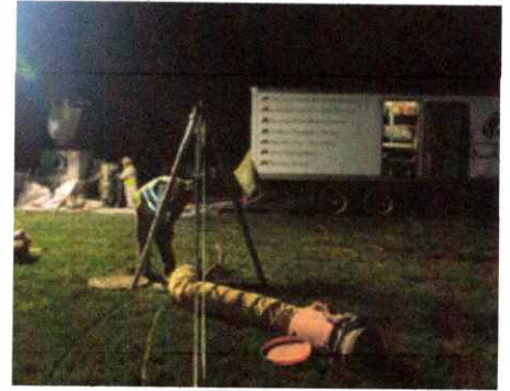
Above ground work on 36" RCP rehabilitation.
