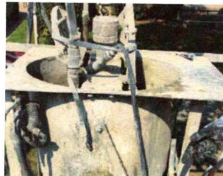
GeoSpray mixed and prepared to send for application.
