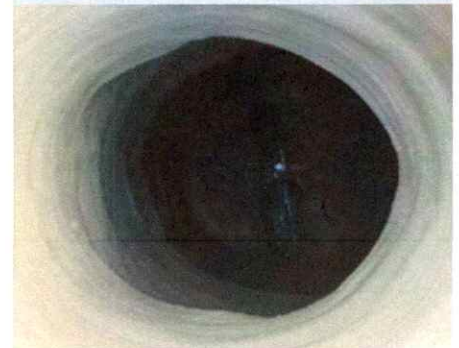
Completed manhole rehabilitation.
