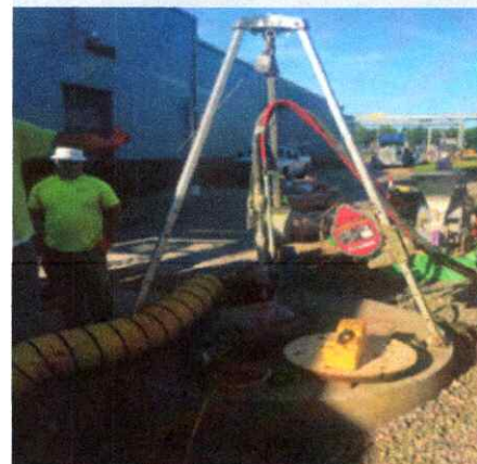
Equipment requires minimal space for manhole rehabilitation using GeoSpray mortar.
