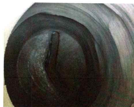
Completed manhole rehabilitation.
