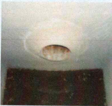
Manhole renewed with GeoSpray geopolymer.
