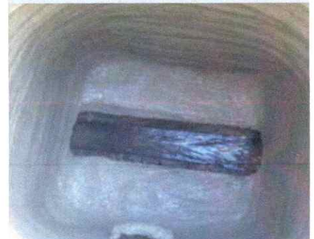
Like-new manhole and bench after GeoSpray mortar application.
