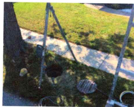
Typical manhole application in right-of-way with tripod set up.
