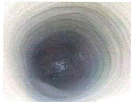
Completed manhole repair.
