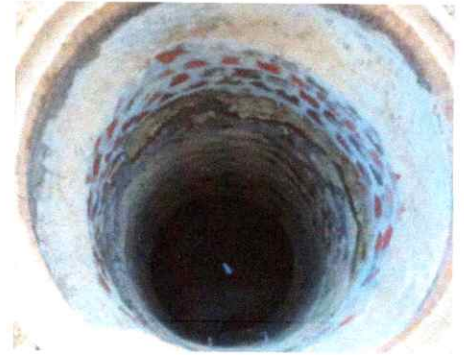
Manhole prior to spraying.
