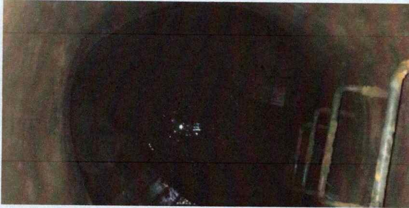
Existing cement manhole.
