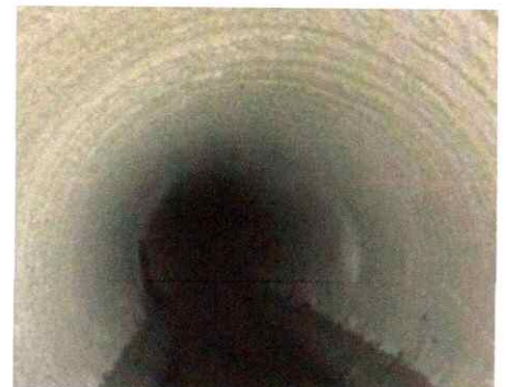
Completed RCP rehab with GeoSpray geopolymer lining.
