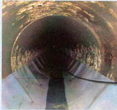
36" folded liner pulled in place.
