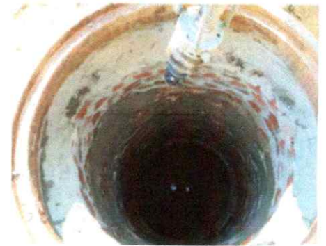
Start of GeoSpray mortar application.
