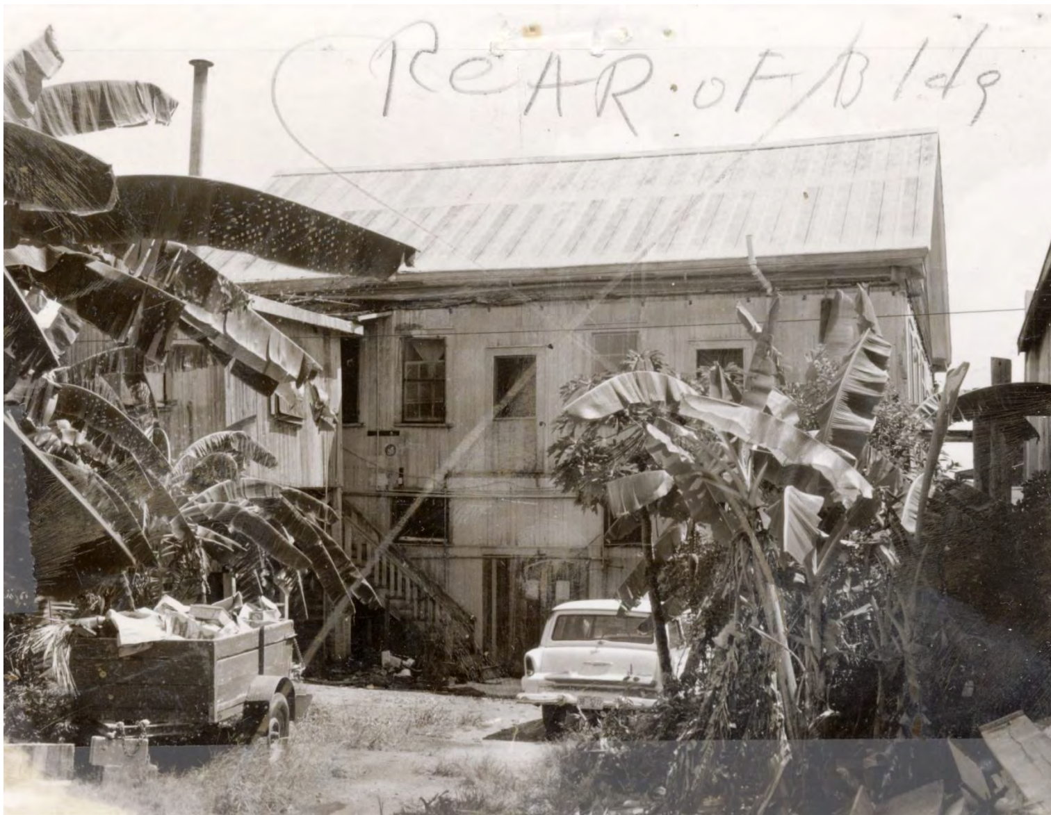
218 Duval Street rear of building circa 1965. Monroe County Library.
