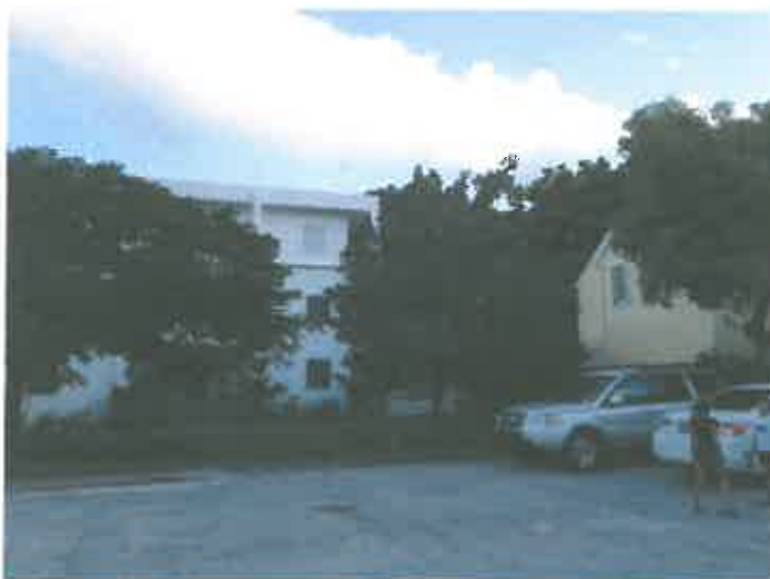
ST. MARY'S GYM WITH CONDOS ON RIGHT BEYOND WALL
