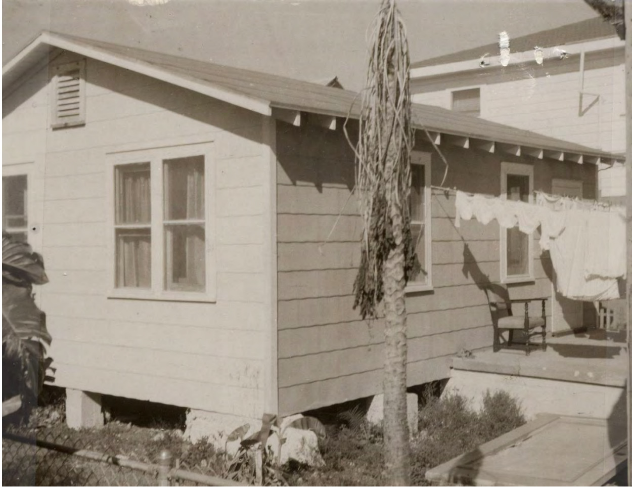
Accessory structure under review circa 1965. Monroe County Library.
