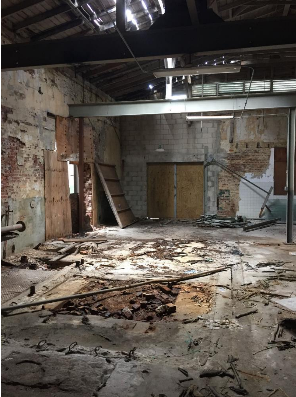
PHOTO 4: Interior of buildings at the Site
