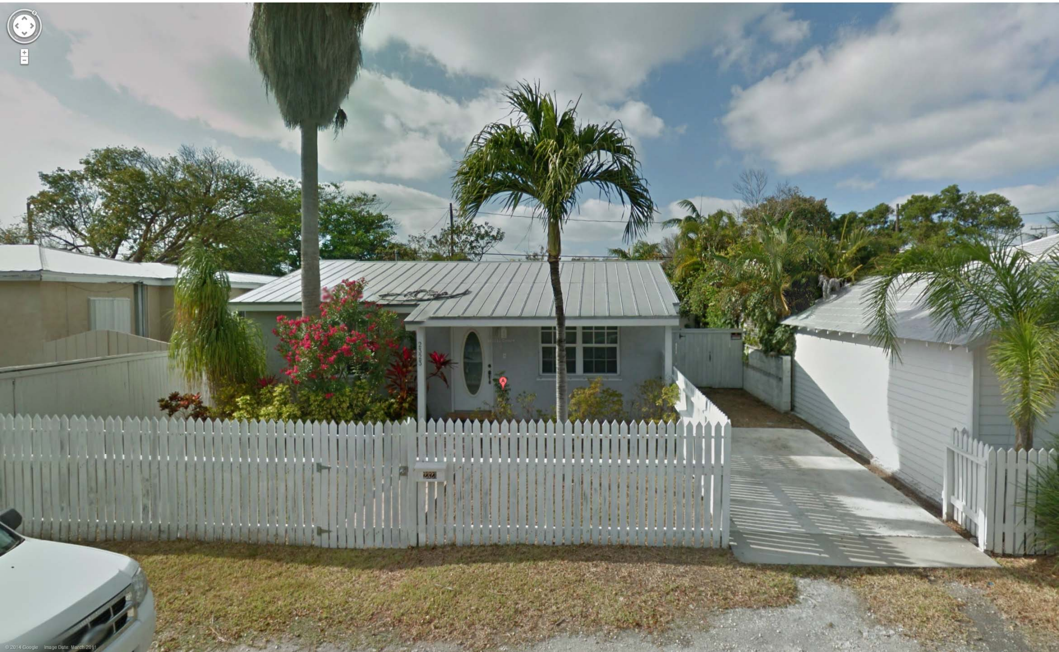
Google StreetView of 2323 Staples Avenue prior to construction of the second floor addition.
