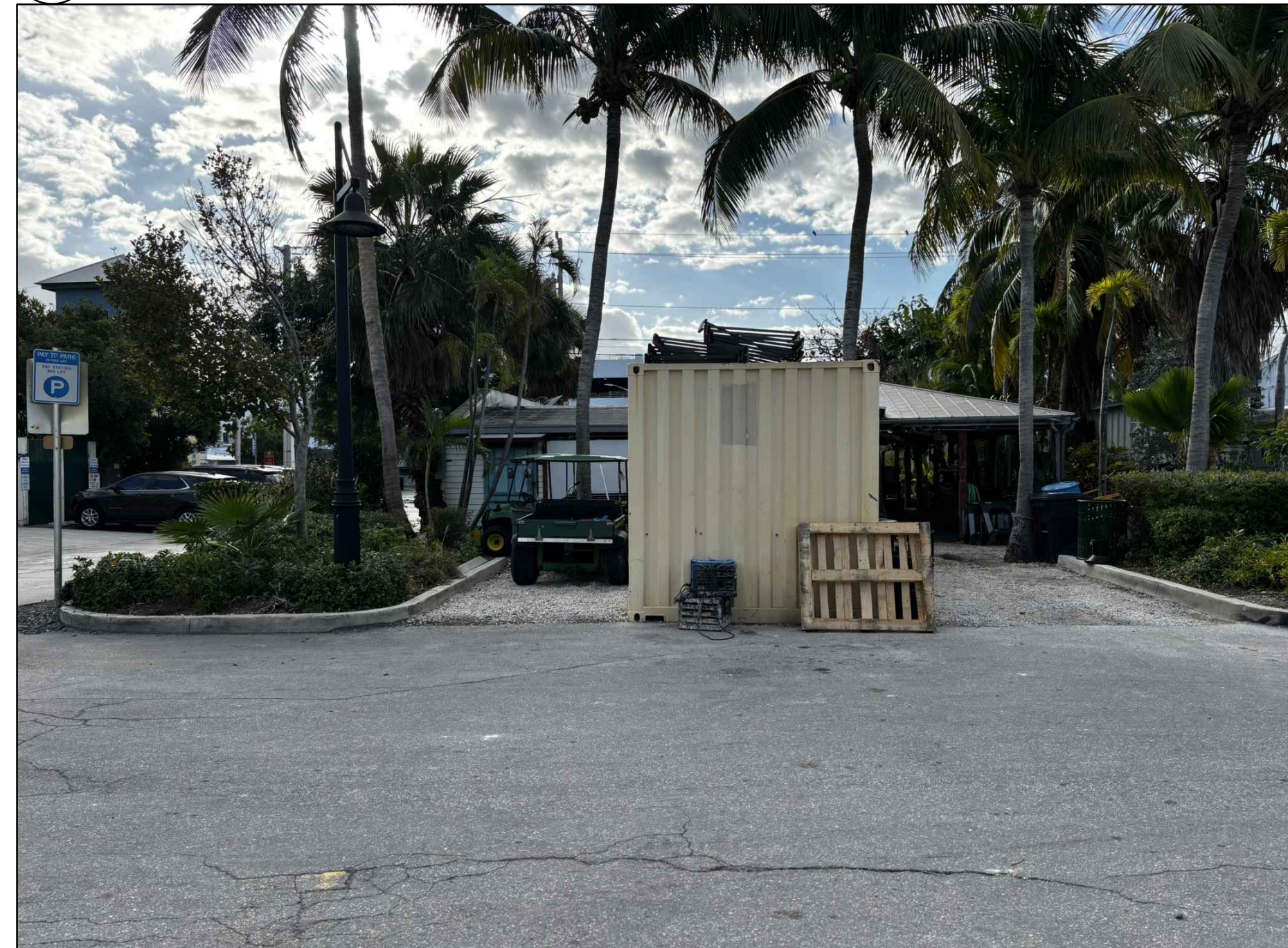
5 VIEW OF THE BACK OF THE BUILDING (EXISTING NORTH ELEVATION) A6 SCALE: N.T.S.
