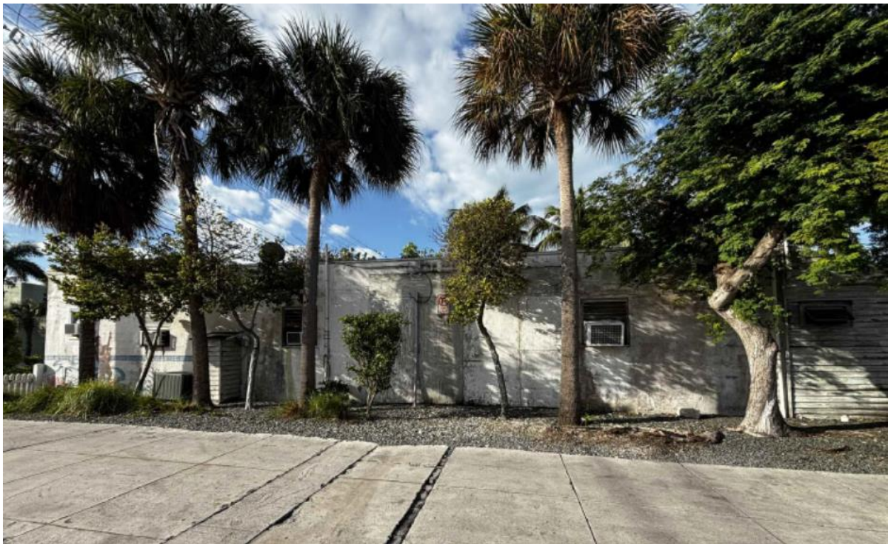
Side elevation of structure.
