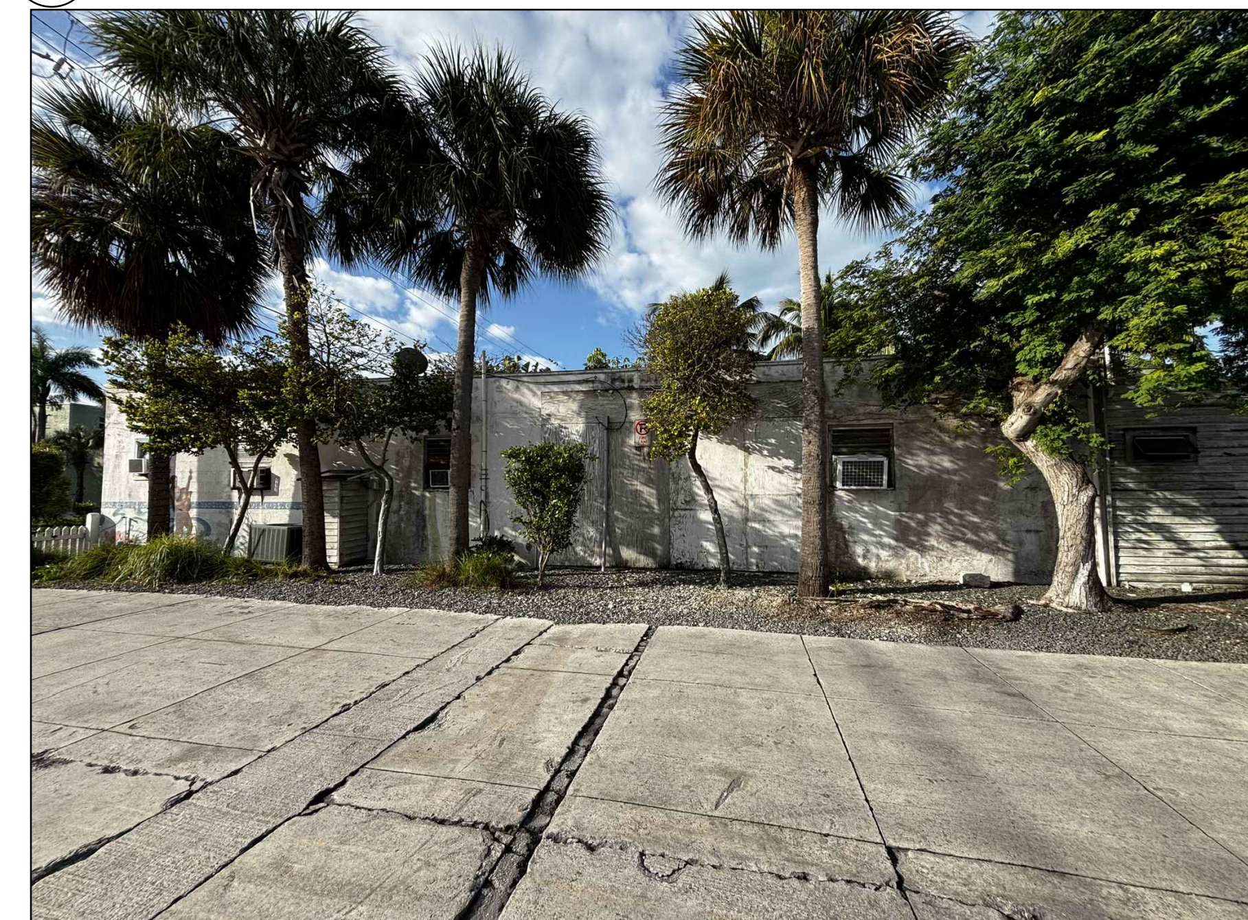
2 VIEW OF THE SIDE OF THE BUILDING (EXISTING EAST ELEVATION) A6 SCALE: N.T.S.
