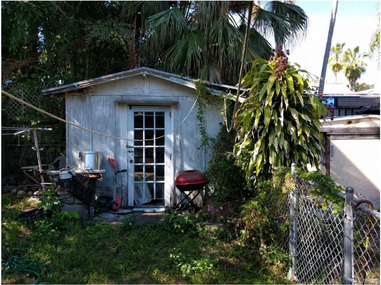
ACCESSORY STRUCTURES AT REAR OF PROPERTY
