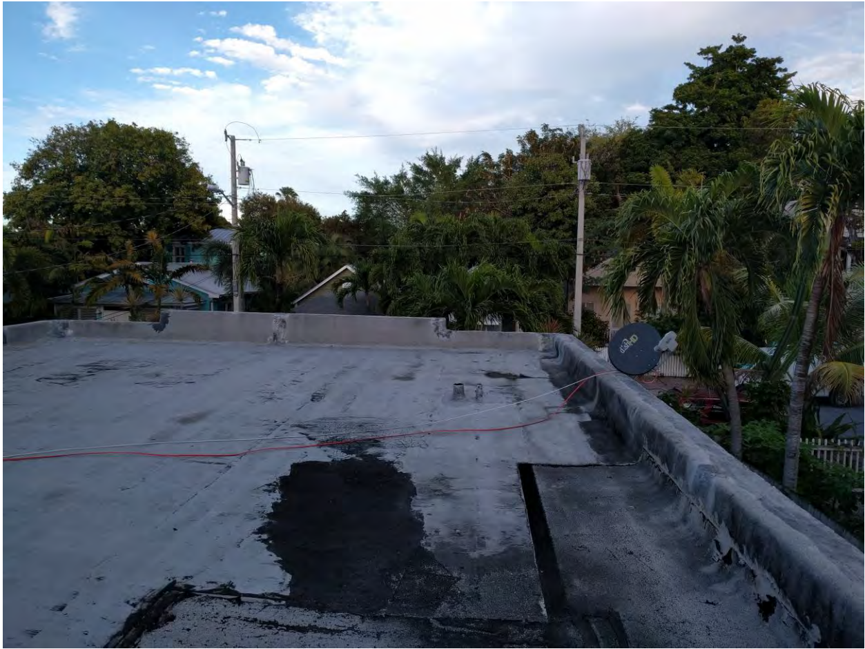
VIEW OF EXISTING ASPHALT FLAT ROOF
