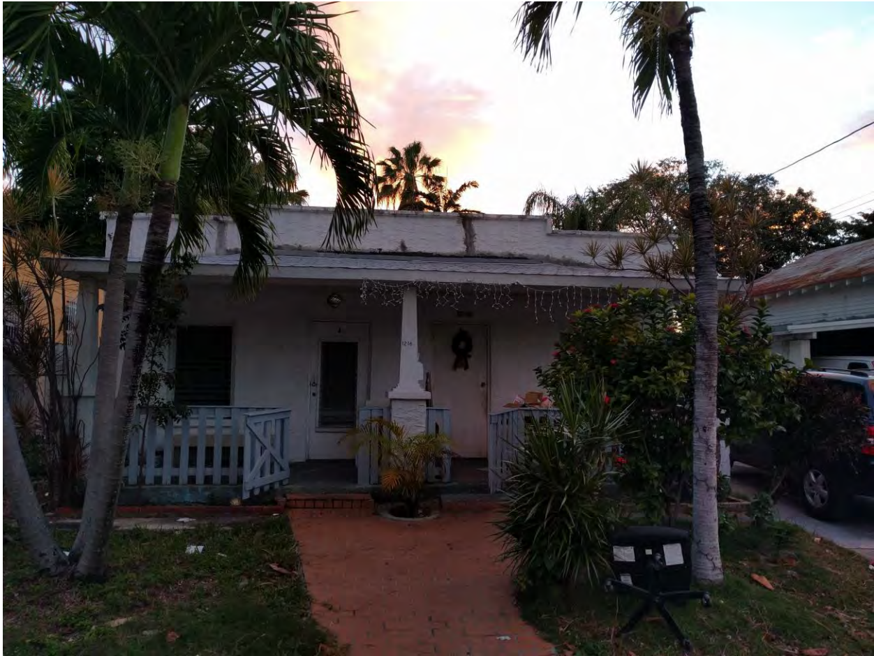
CURRENT VIEW – FRONT FAÇADE
