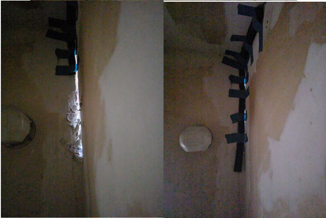
DETERIORATED WALL CONDITION (SEPARATION)
