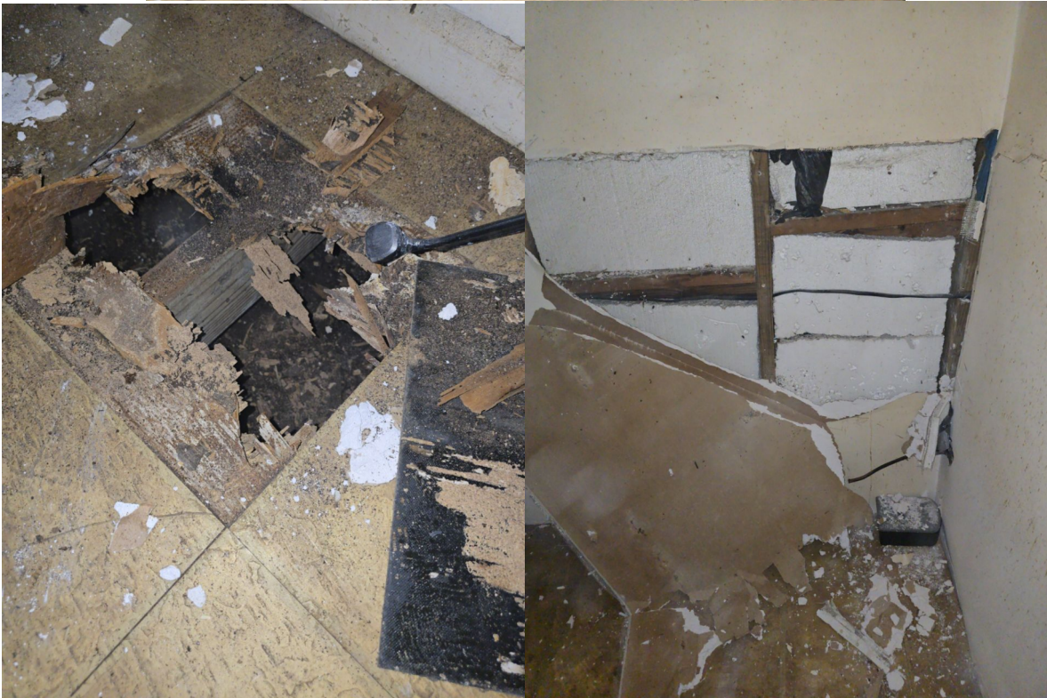
DETERIORATED FLOOR FRAMING & SHEATHING
