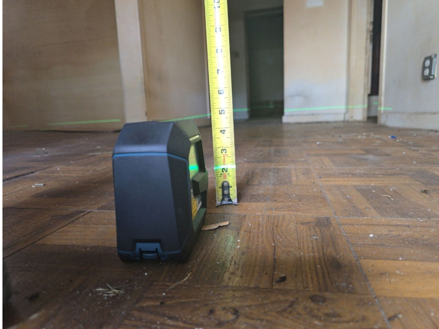
UNLEVEL FLOOR (SUNKEN FOUNDATION & FRAMING)
