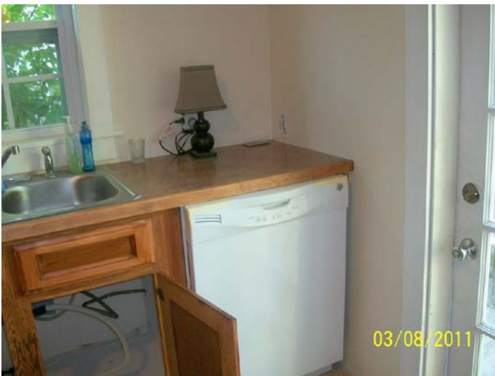
New electrical for dishwasher wired directly
