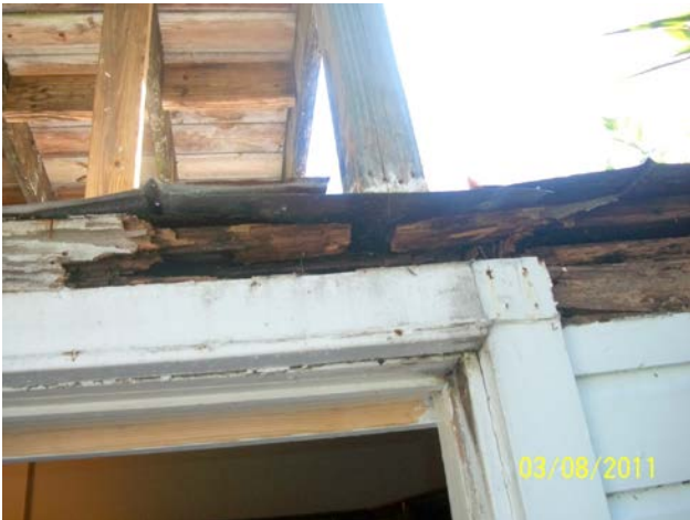
Back balcony standing on rotten roof
