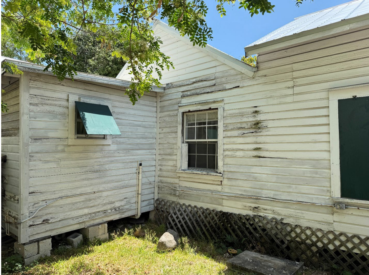
Figure 6 – North Side of house – Sawtooth and Flat Roof Additions in scope
