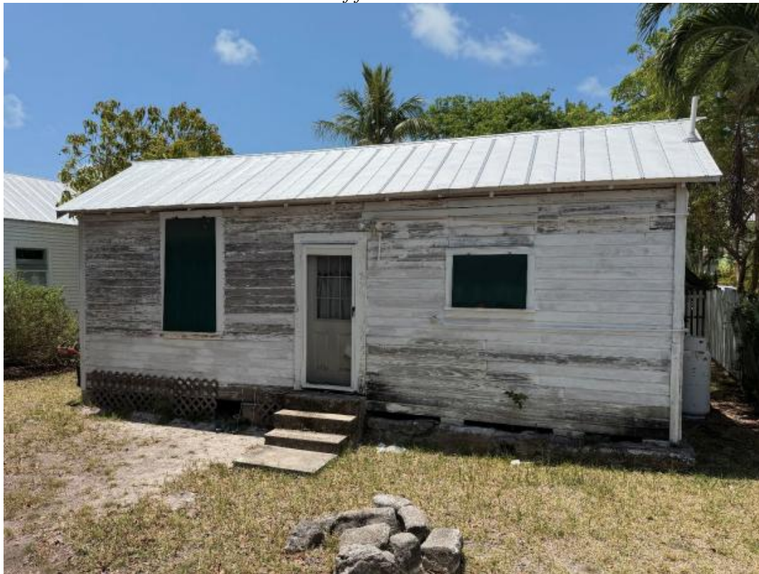
Photo of rear elevation.
