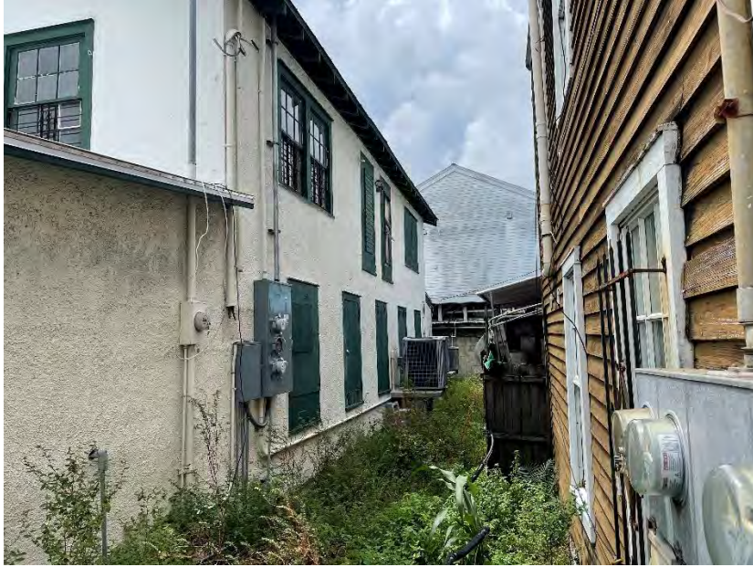
Rear of Charles Street structure adjacent to 4 Charles Street
