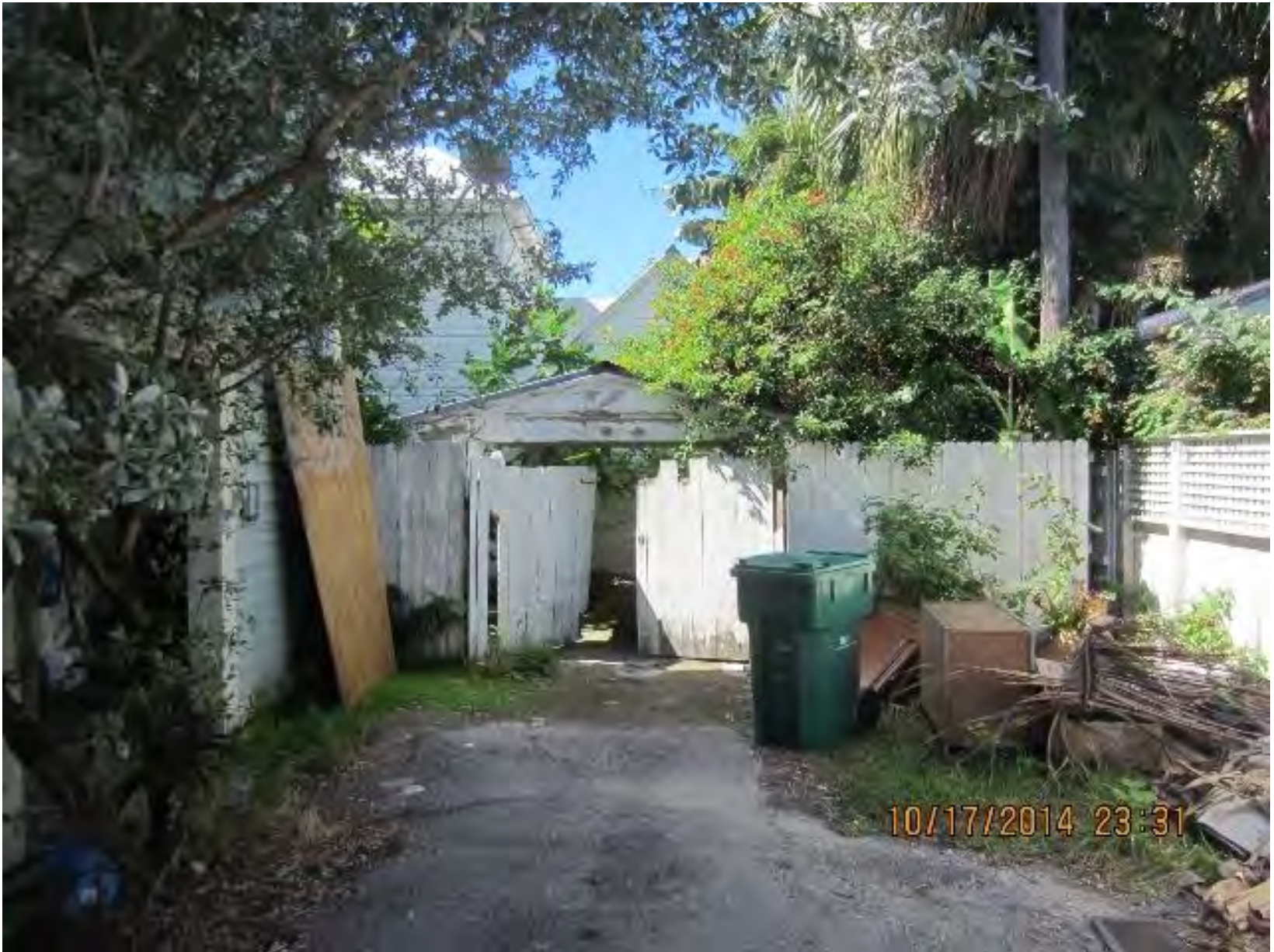
View of rear of house from Stickney Lane
