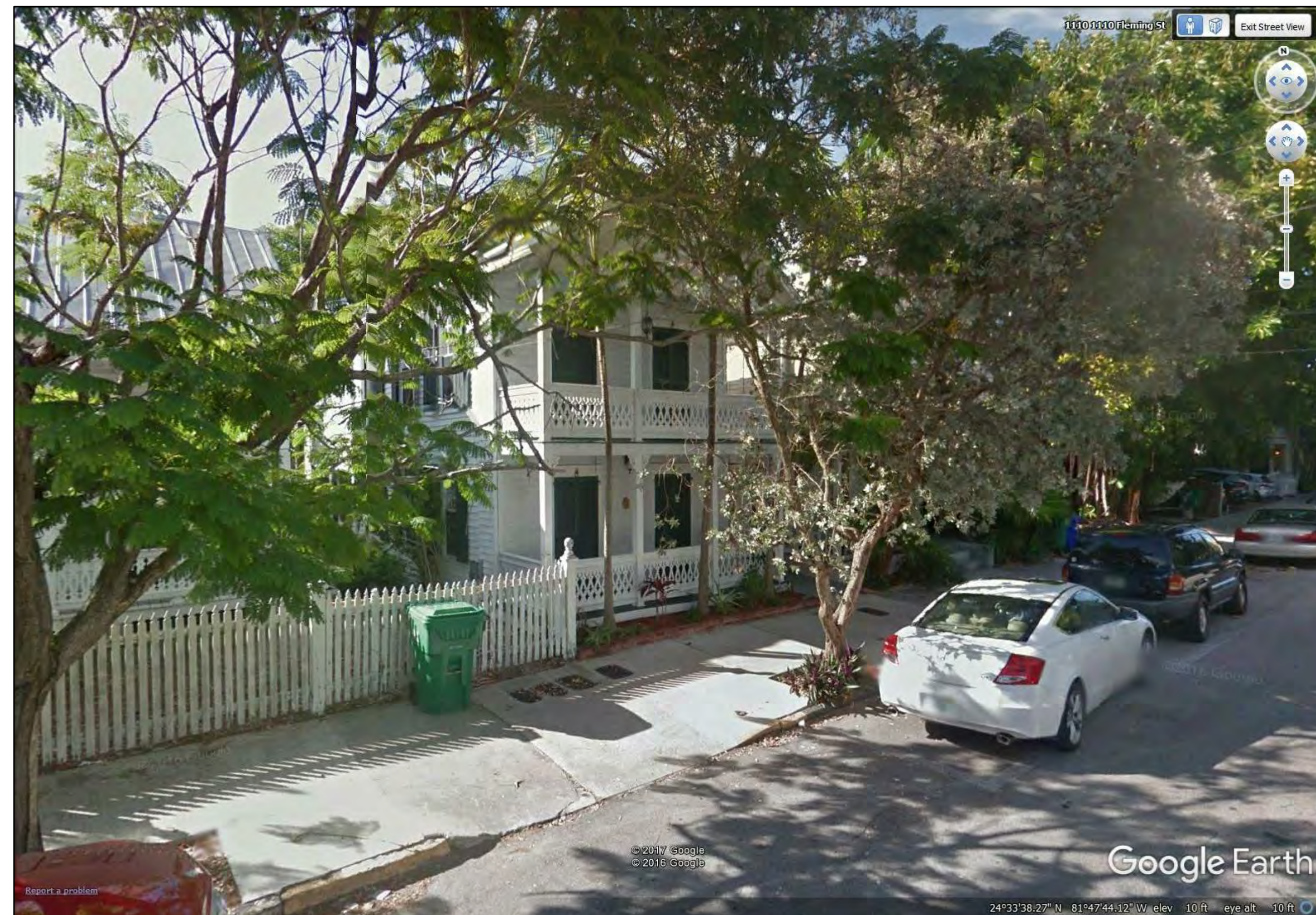
2 ADJACENT PROPERTY TO THE EAST
