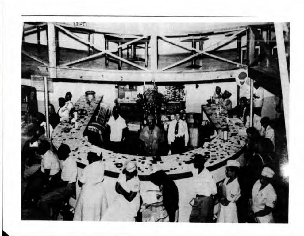
The original horseshoe-shaped bar is seen in this photo, date unknown. The bar is topped with broken Cuban tile set in mortar. The bar will be reconstructed when funds allow.
