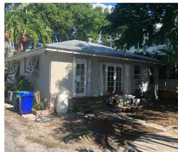
6 PHOTO OF 520 GRINNELL WEST EXTERIOR ELEVATION
