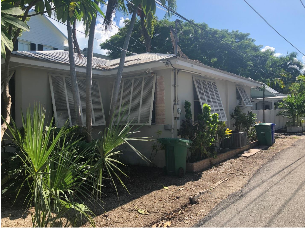
Photo of 520 Grinnell North Exterior Elevation.
