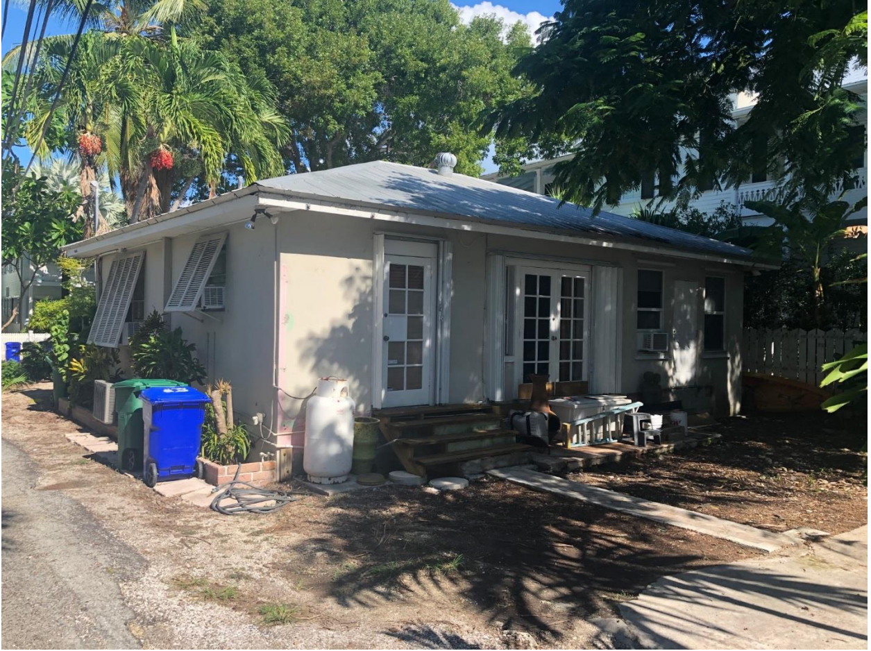
Photo of 520 Grinnell West Exterior Elevation.
