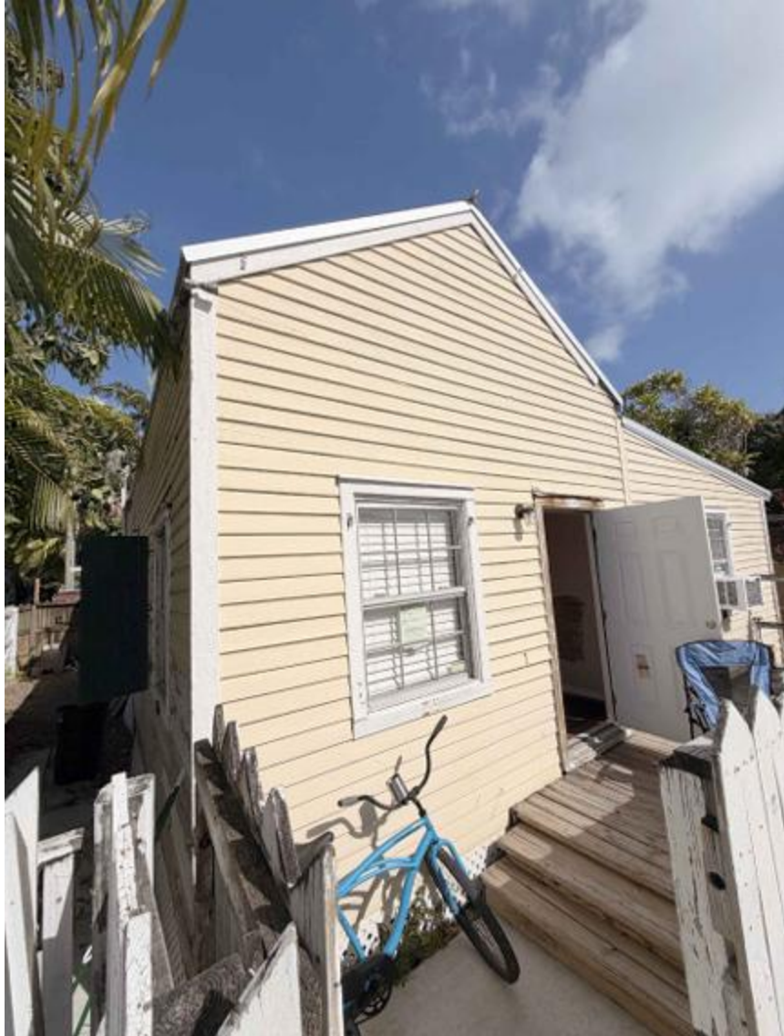
Photo of property under review, view from Virginia Street.
