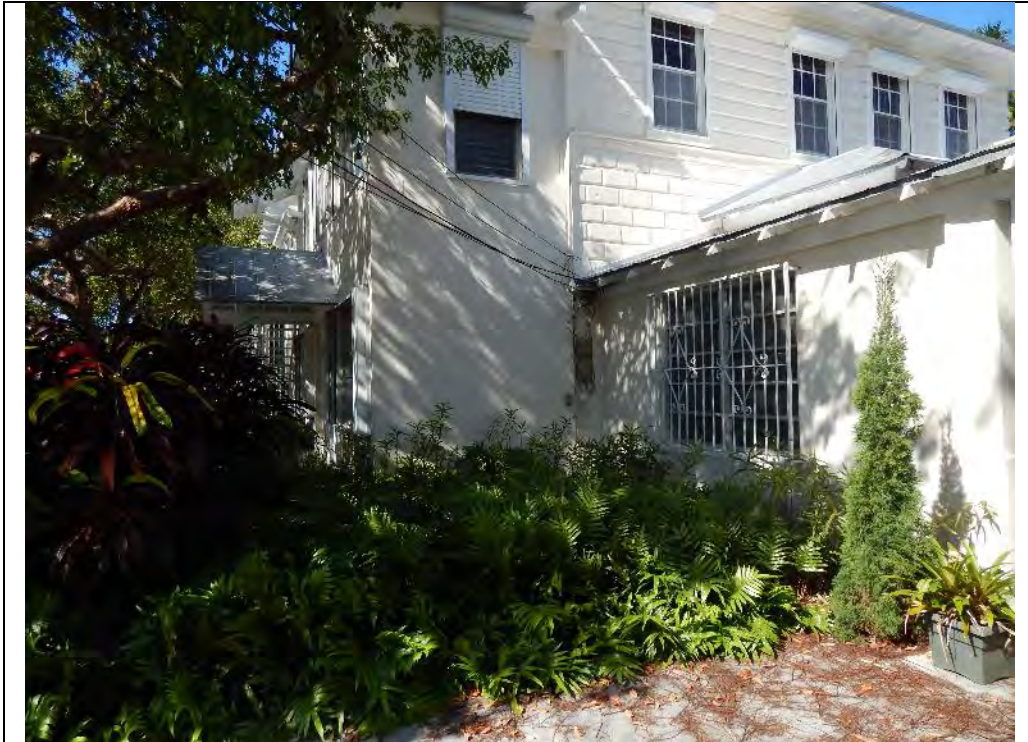
3. 1019 Flagler. View from east driveway.
