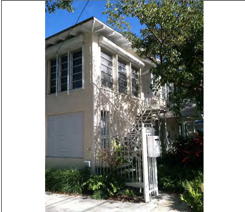
5. 1019 Flagler. View from carport / west driveway.
