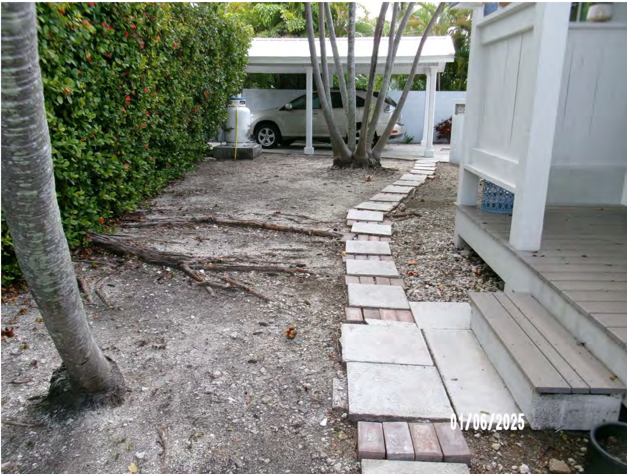
Photo showing root zone area in relation to structure.
