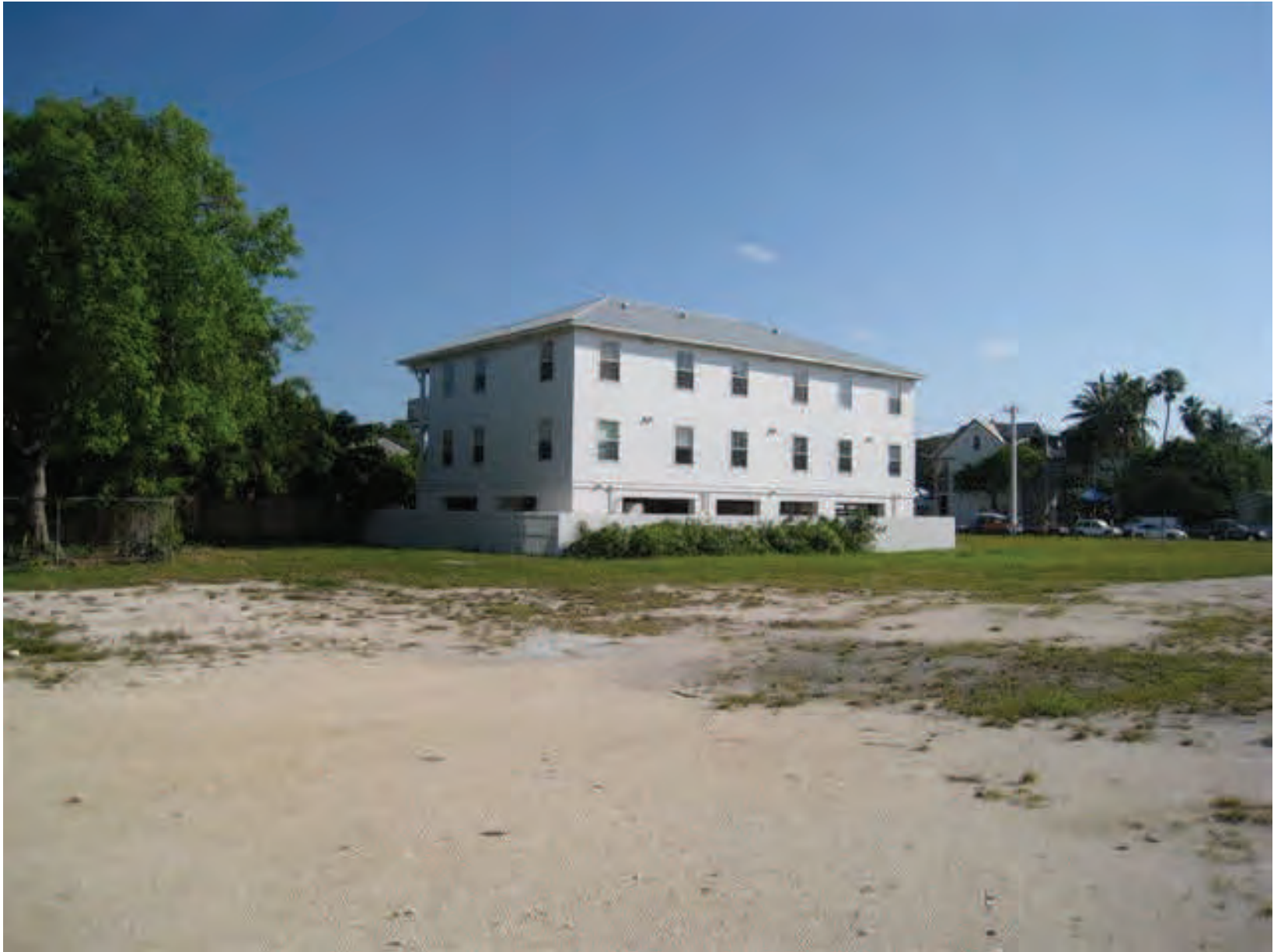
VIEW FROM SITE LOOKING SOUTH TO APARTMENT
