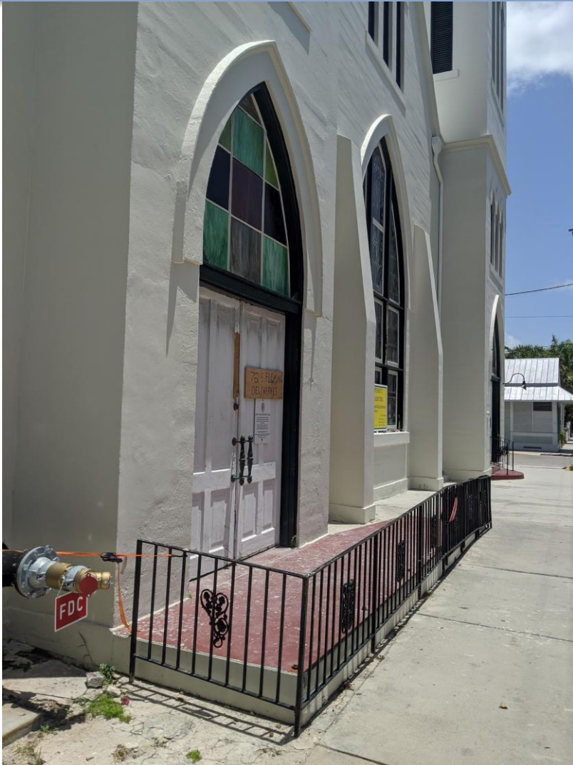
Existing Fleming Street ADA ramp
